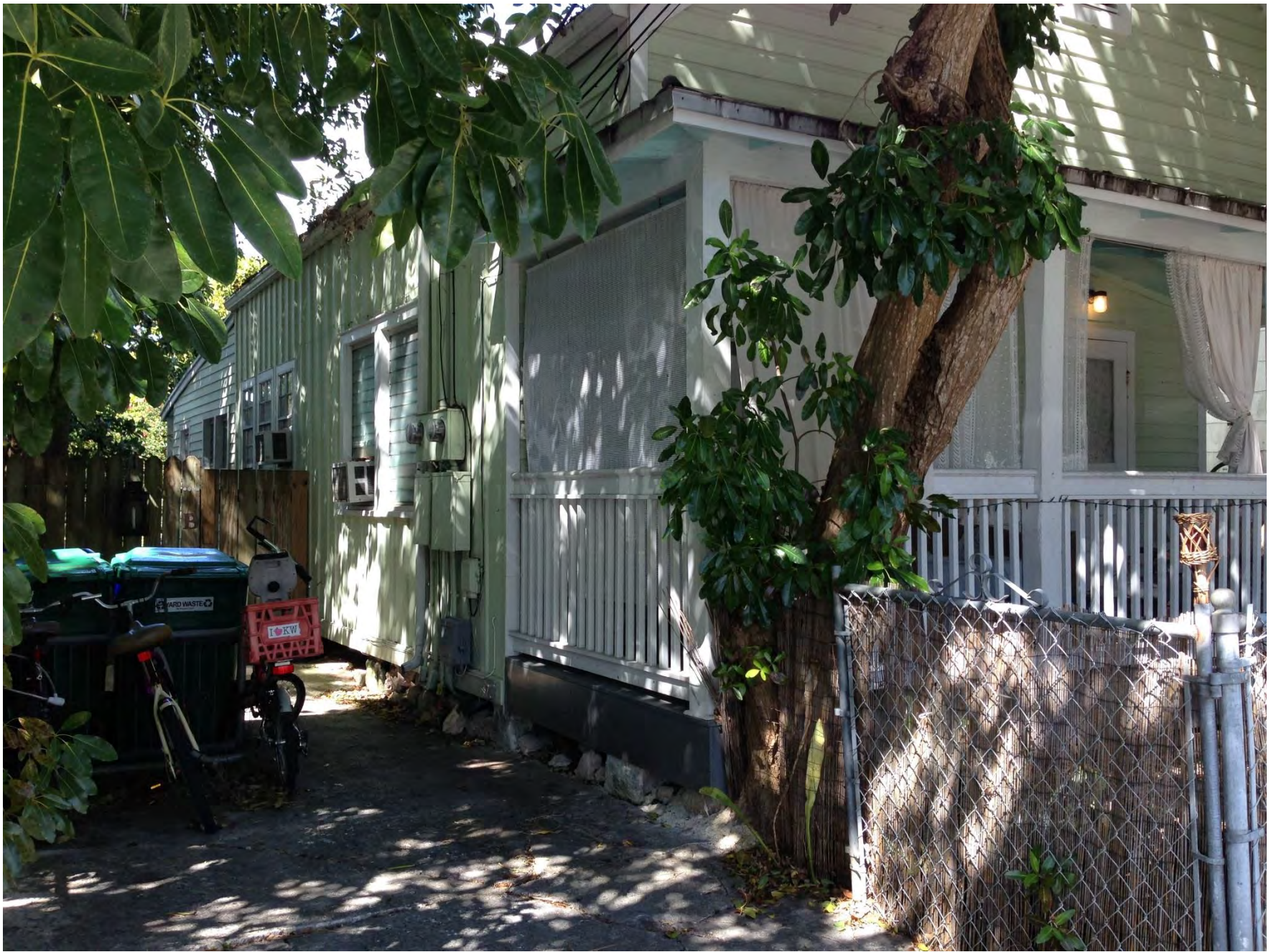
Board and batten siding on side of 1307 Newton.
