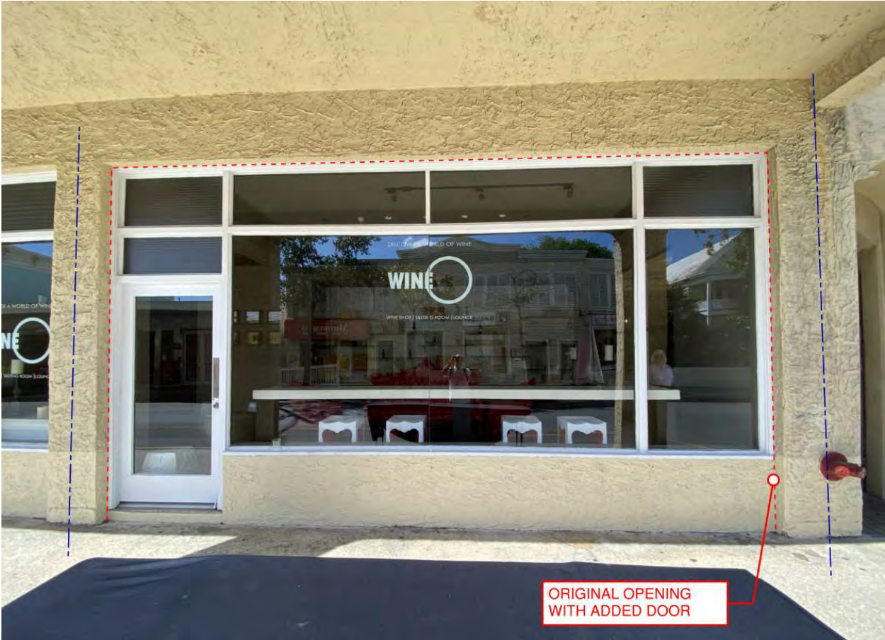
Bay 7 – existing conditions
