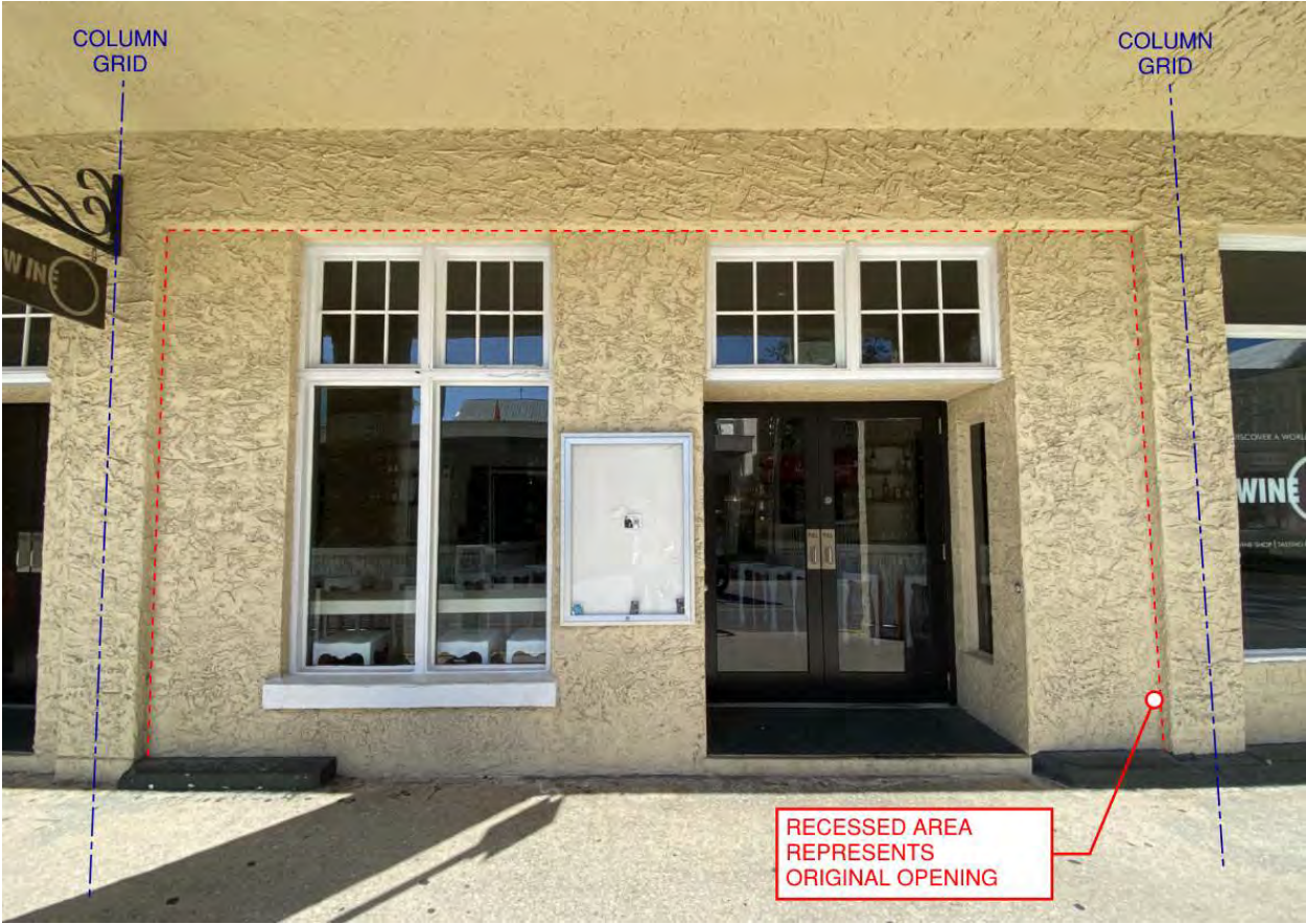
Bay 5 – existing conditions
