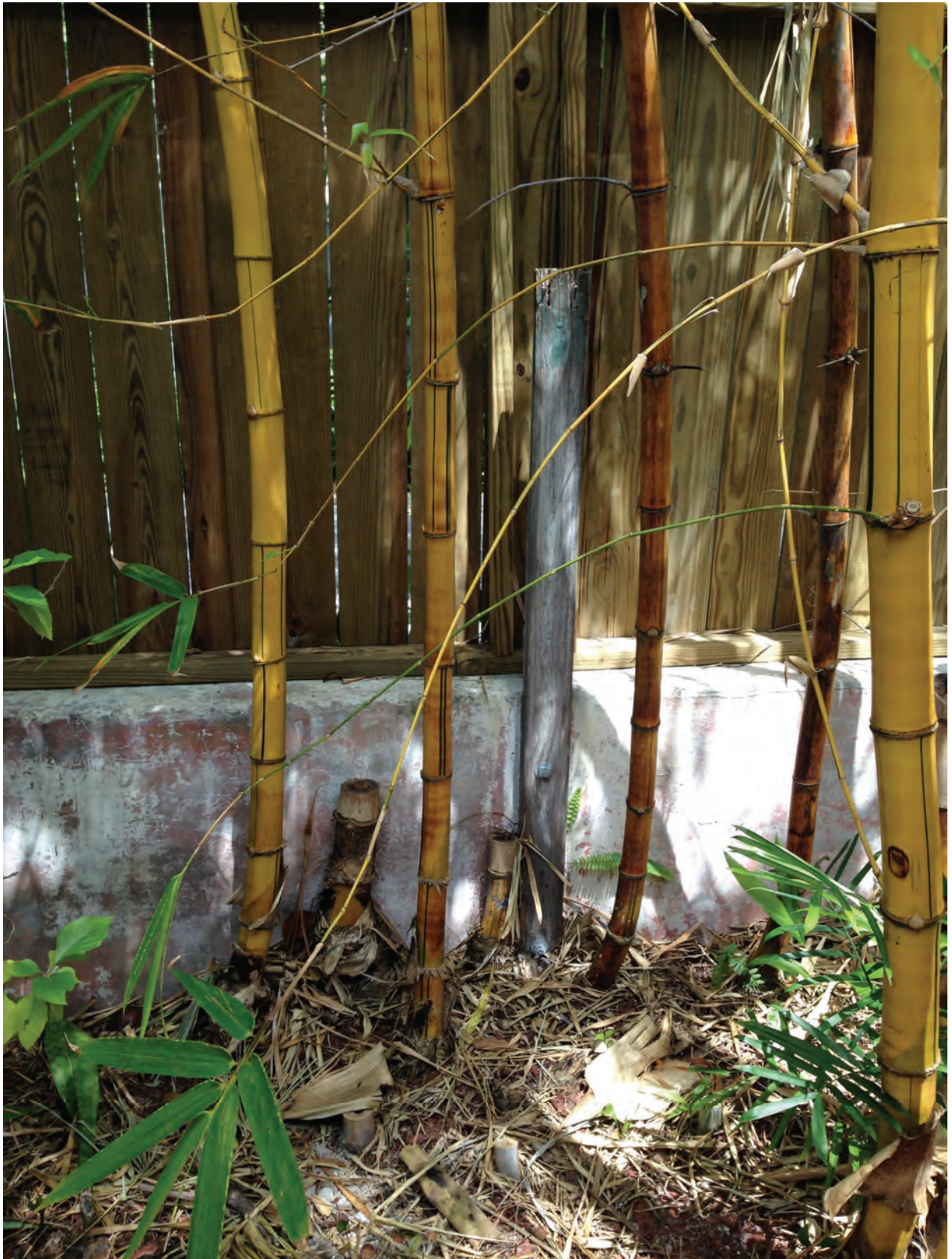
907 Frances (view from inside the yard) Concrete wall
