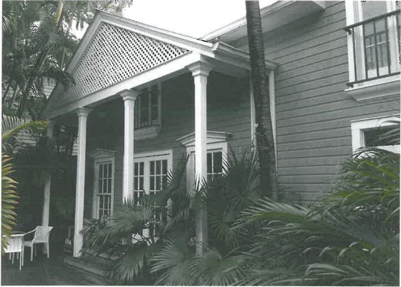
This is a porch addition to the Pool House, 1989. The new porch on the rear of Main House will be similar.
