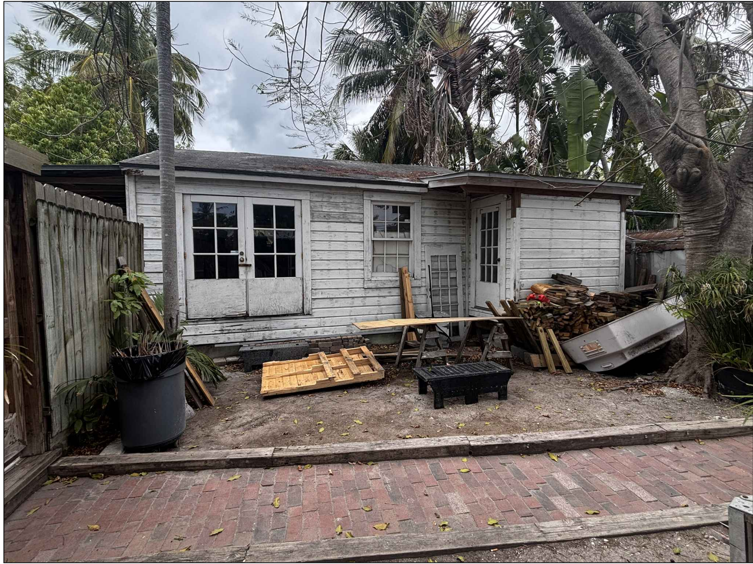
1 A6 VIEW FROM SOUTH SIDE OF THE PROPERTY SCALE: N.T.S.
