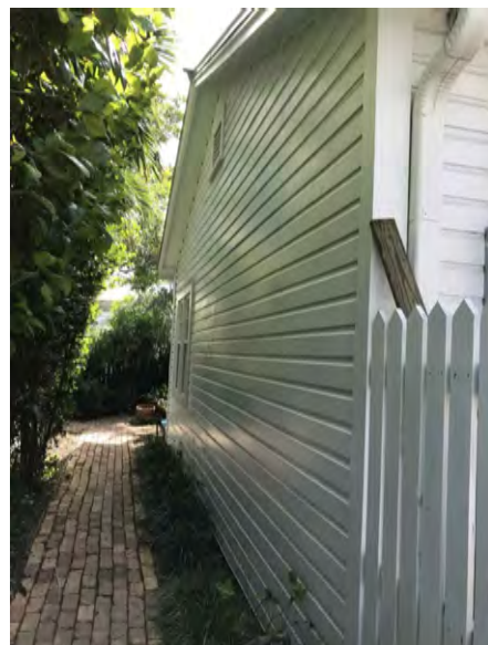
EXISTING N. SIDE OF HOUSE FROM FRONT
