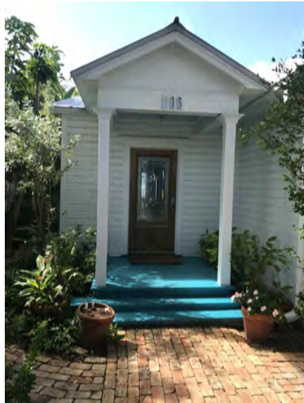
EXISTING FRONT PORCH
