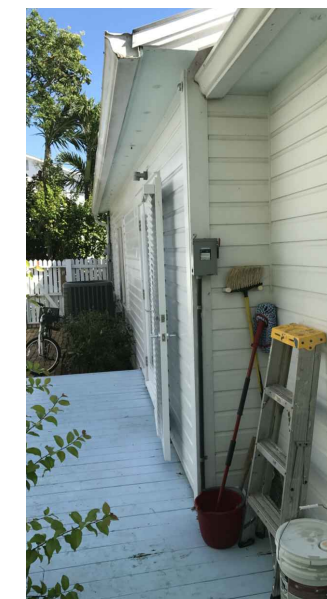
EXISTING N. SIDE OF HOUSE FROM REAR
