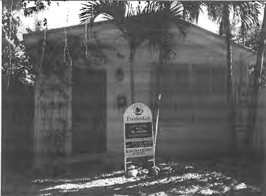
Front View & Electric Panel 11/1/13
