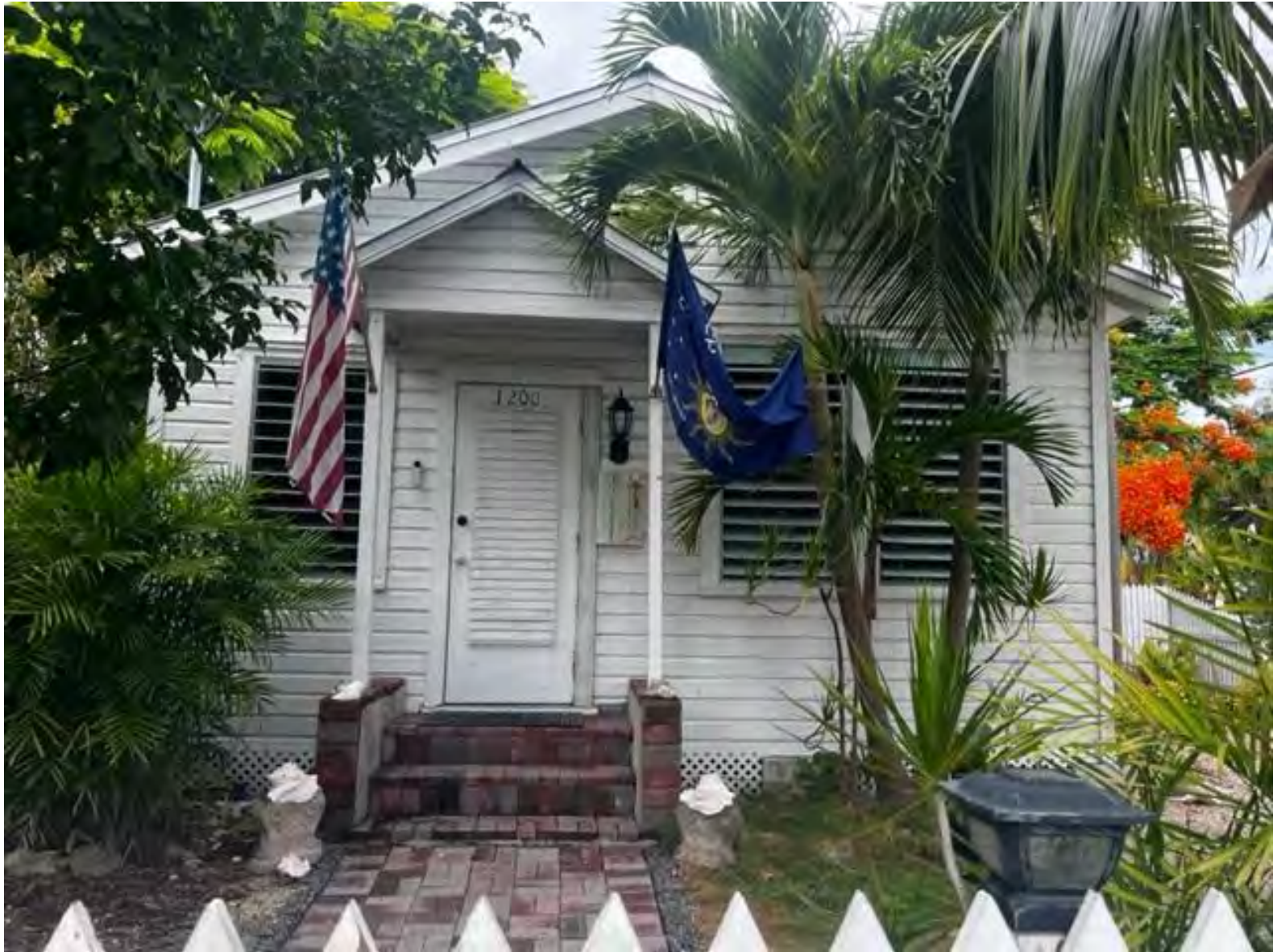
Front elevation facing Margaret Street.
