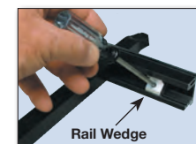
Tightening rail wedge on shortened section.
