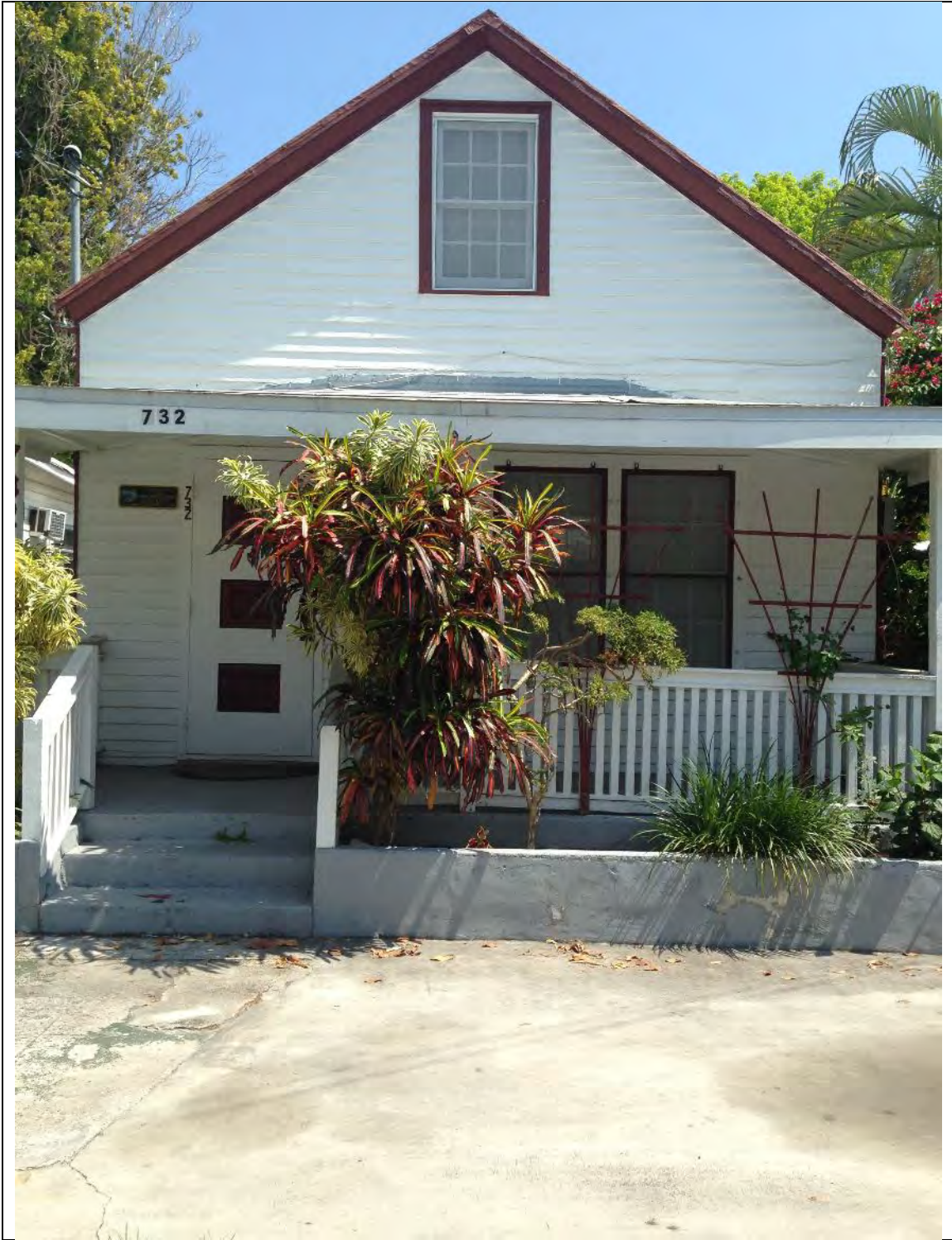
1. 732 Poorhouse Lane. View from the street.
