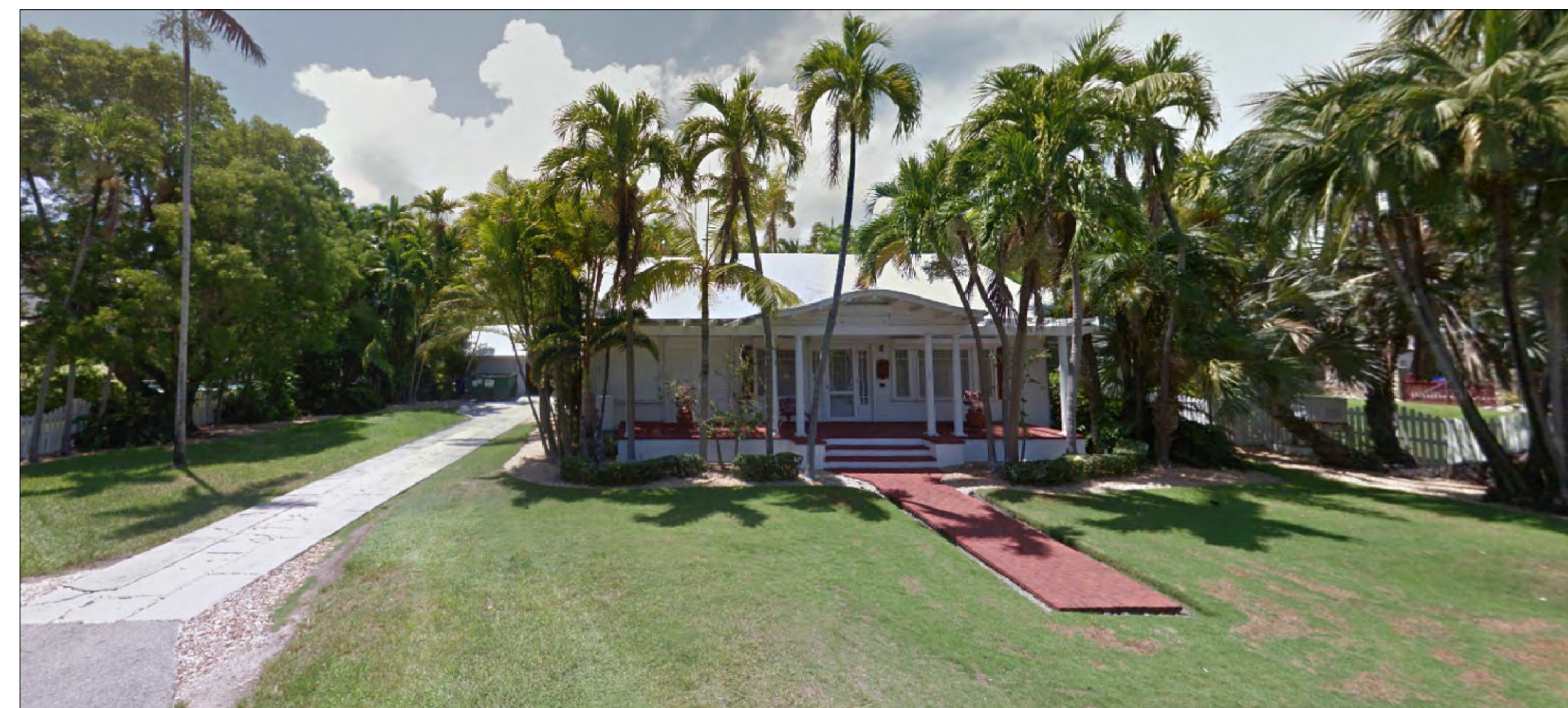
STREET VIEW (FROM WASHINGTON STREET) 2015
