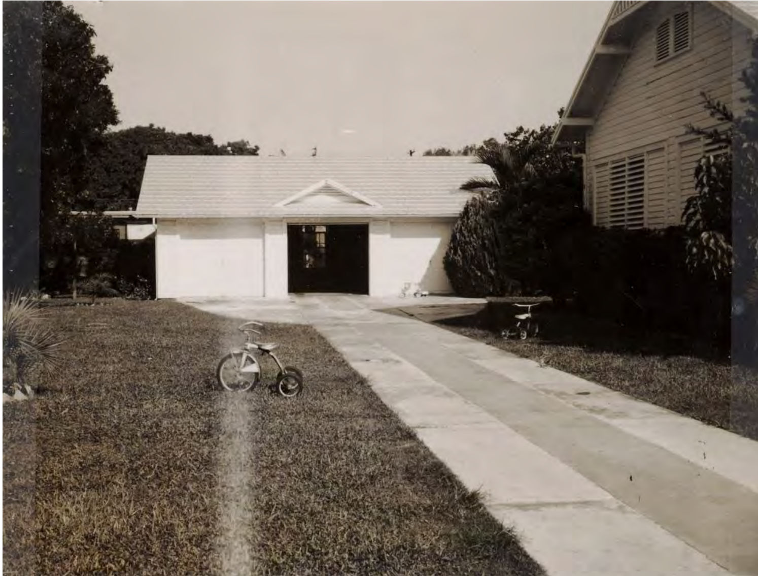
#1021 Washington Street garage circa 1965. Monroe County Library
