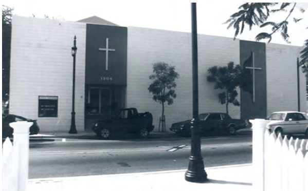
Same view prior to removing 1960's addition that obscured the Sanctuary. Sanctuary windows were intact behind the addition, but the front porch required reconstruction. Note the Sanctuary roof above the 1960's addition.
