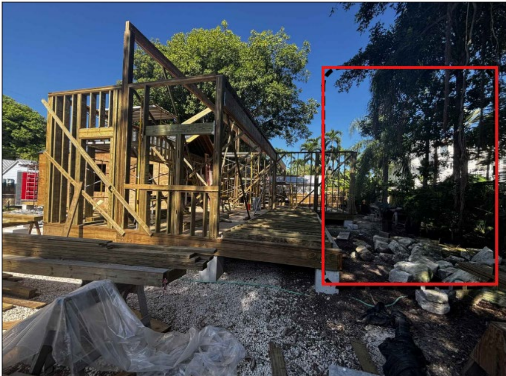
Current Photo of House Under Review.
