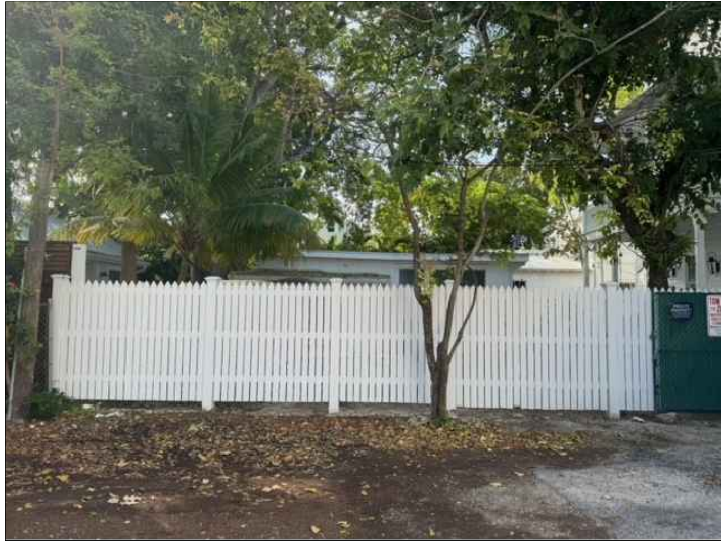
5 VIEW FROM NEIGHBORING PROPERTY (EXISTING NORTH ELEVATION) A7 SCALE: N.T.S.
