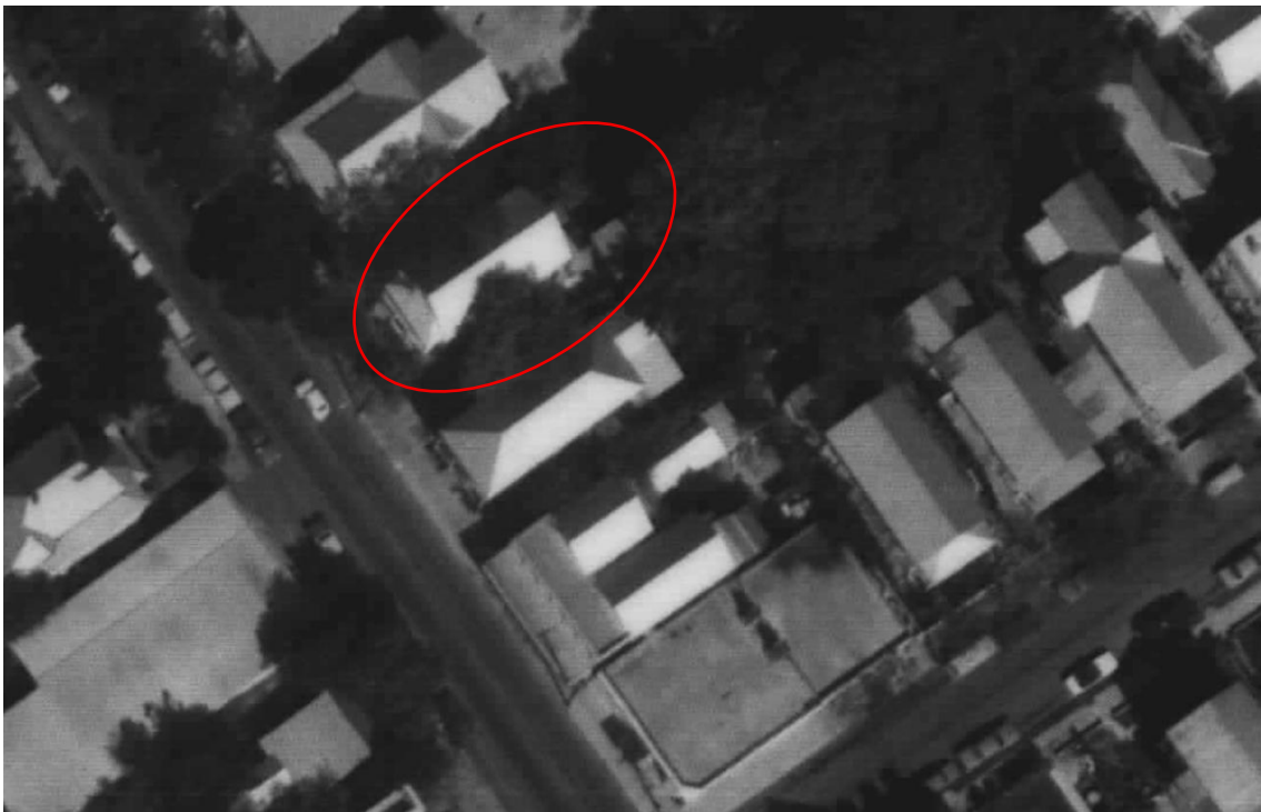
1972 aerial photo showing dwelling unit in rear.
