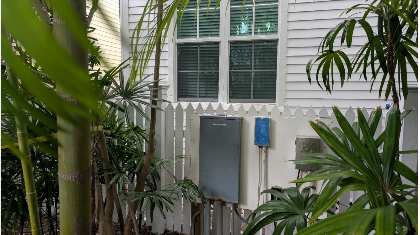
Photo showing current fence between 328 Whitehead Street and neighboring property.
