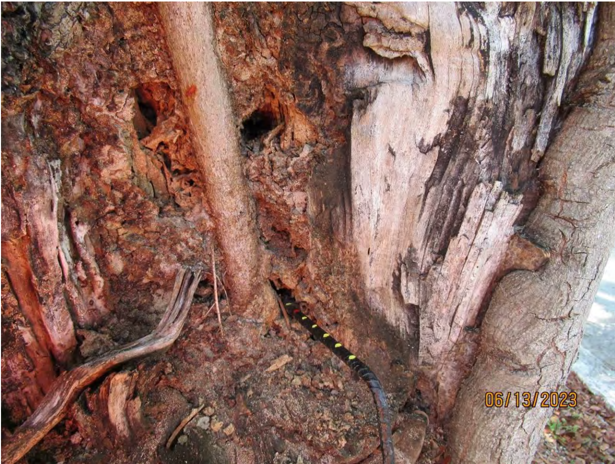
Photo showing probe in right side of decay area (10”).
