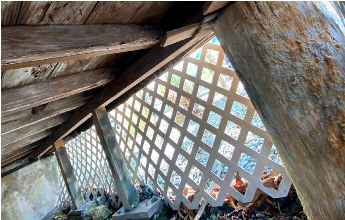
Figure 14. Addition to main building – Heavy damage of wood frame floor system. Perimeter sill beam is completely gone, and floor is supported by temporary shoring. Inadequate repairs of floor joists.
