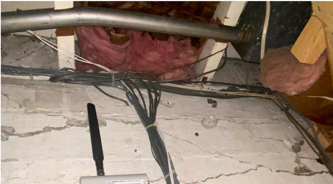
Figure 12. Main Building - Interior view with damaged tie-beam. Misc. damage to roof rafters by electrical conduit pipe.
