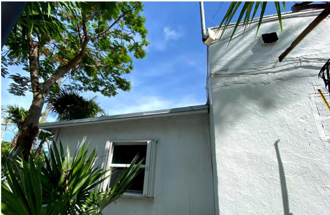
Figure 3. Partial Rear Elevation. Visible concrete damage – cracks along tie-beam.
