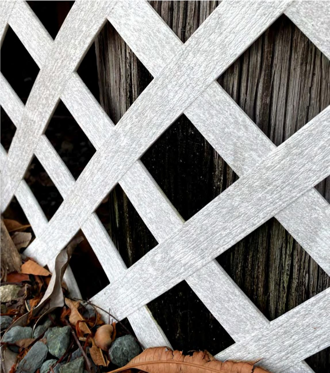
Figure 17. Damaged failing timber pile piers. In need of replacement.
