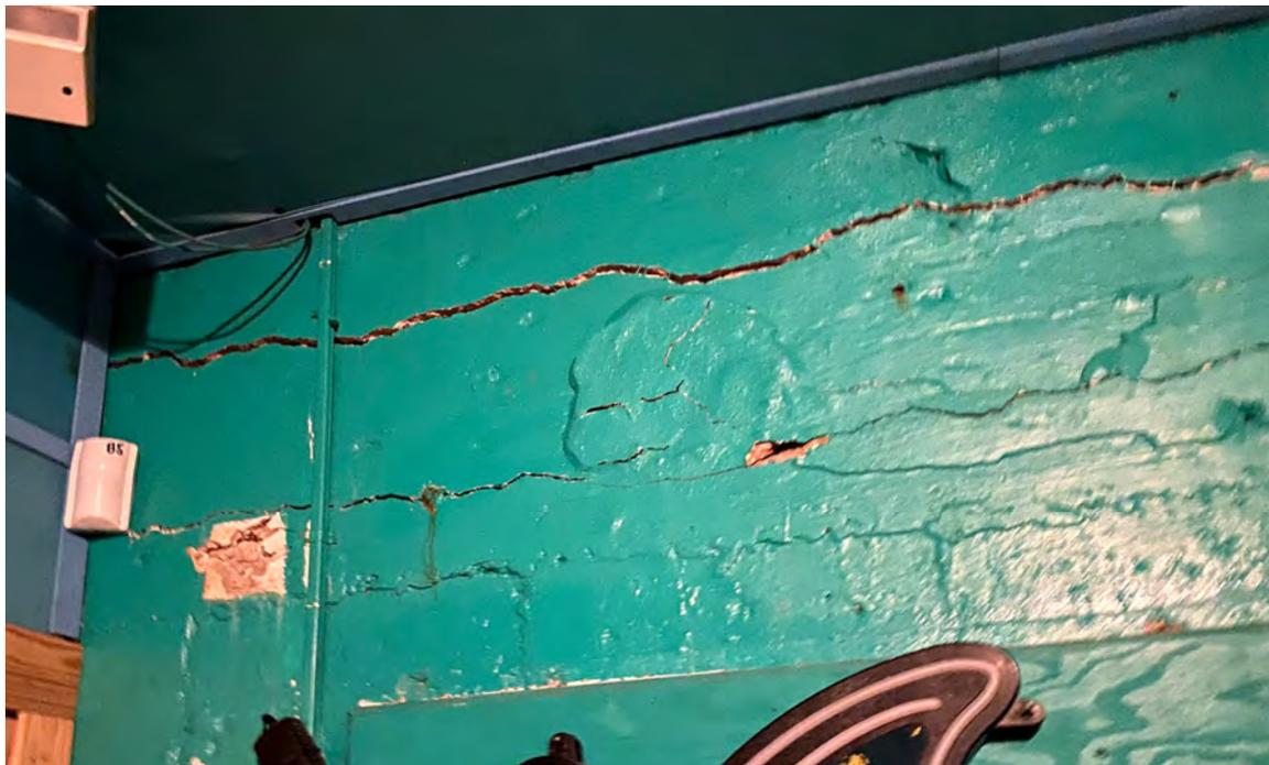
Figure 9. Heavy concrete damage, damaged tie beam (interior of the main building). Please note that on interior the cracks were not patched and are fully open.
