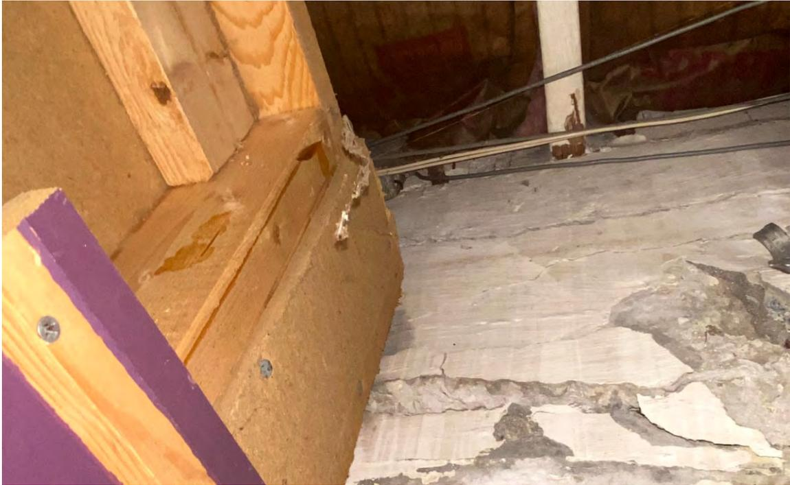
Figure 13. Main Building - Interior view with failing tie-beam.
