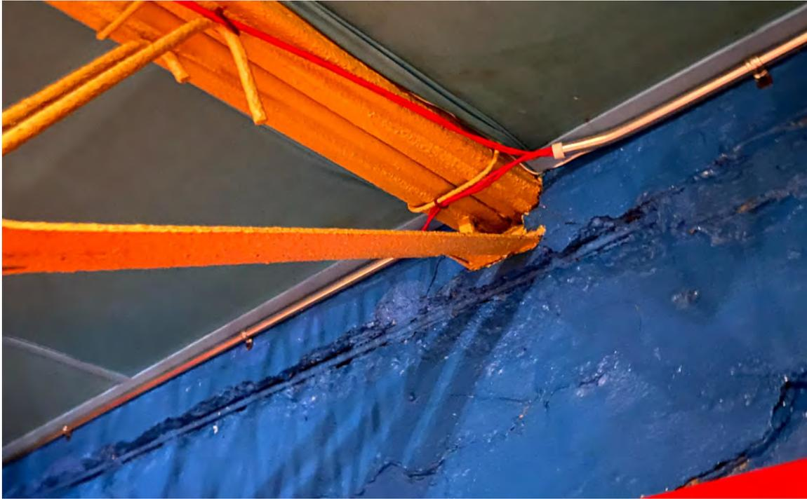
Figure 10. Main Building - Interior view with damaged top of tie-beam at bar joist support. The delaminating (spalling) concrete cover was removed and rebar painted.
