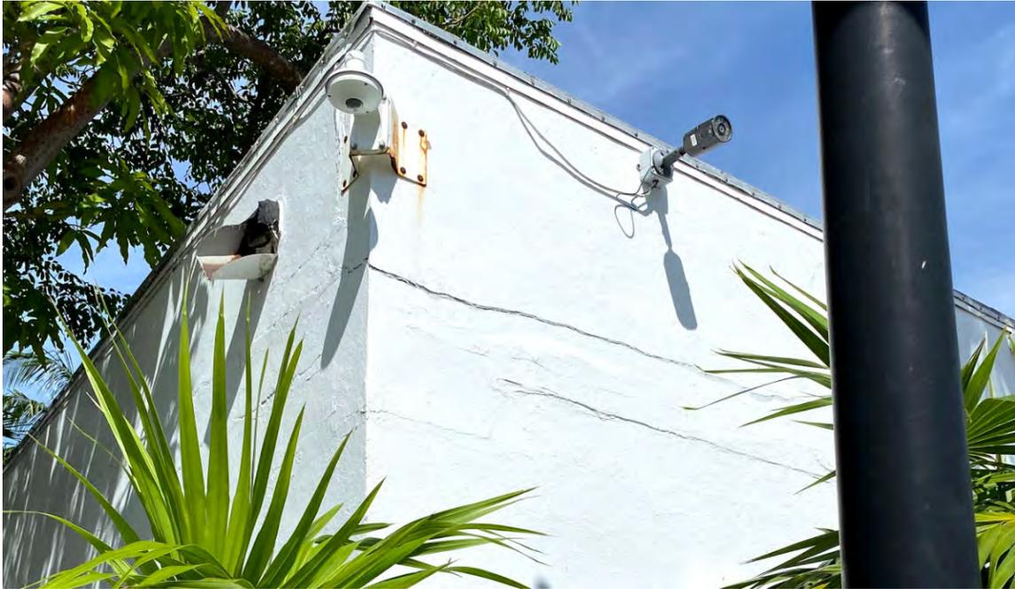
Figure 4. Partial left side elevation. More cracks in the tie-beam.
