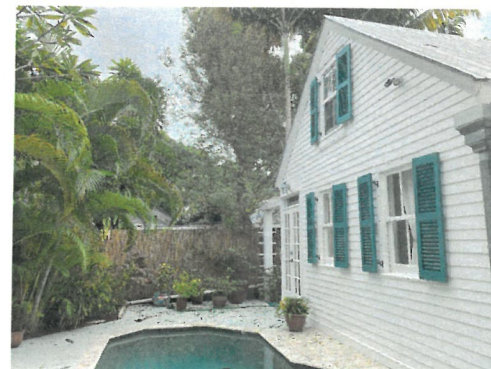
EXISTING PHOTO (PARTIAL REAR ELEVATION) SCALE: NTS
