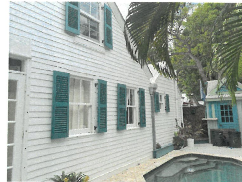
EXISTING PHOTO (PARTIAL REAR ELEVATION) SCALE: NTS
