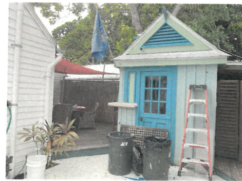
EXISTING PHOTO AREA OF PROPOSED ROOF (PARTIAL REAR ELEVATION) SCALE: NTS
