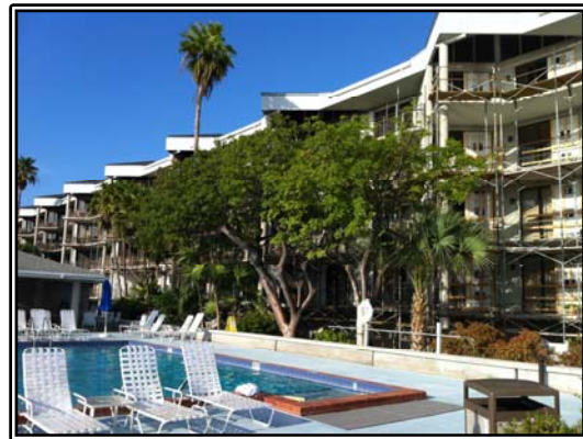
1800 Atlantic Current Work in Progress
