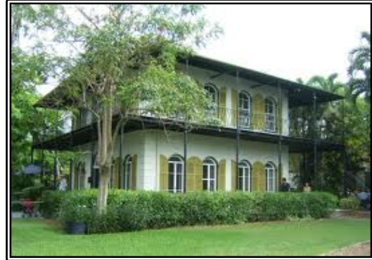
The Hemingway Museum ADA retrofit
