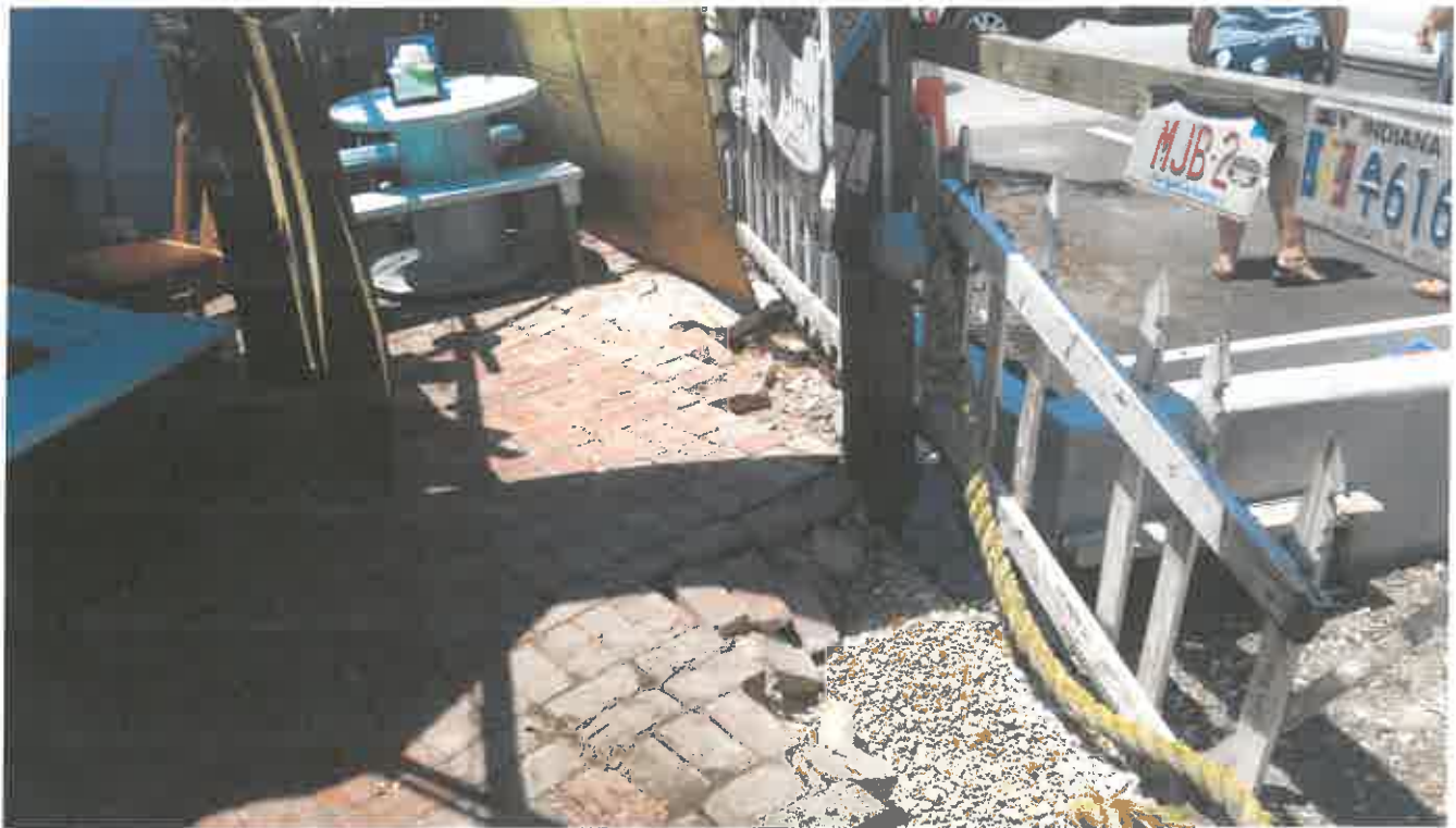
damage inside of dining area
