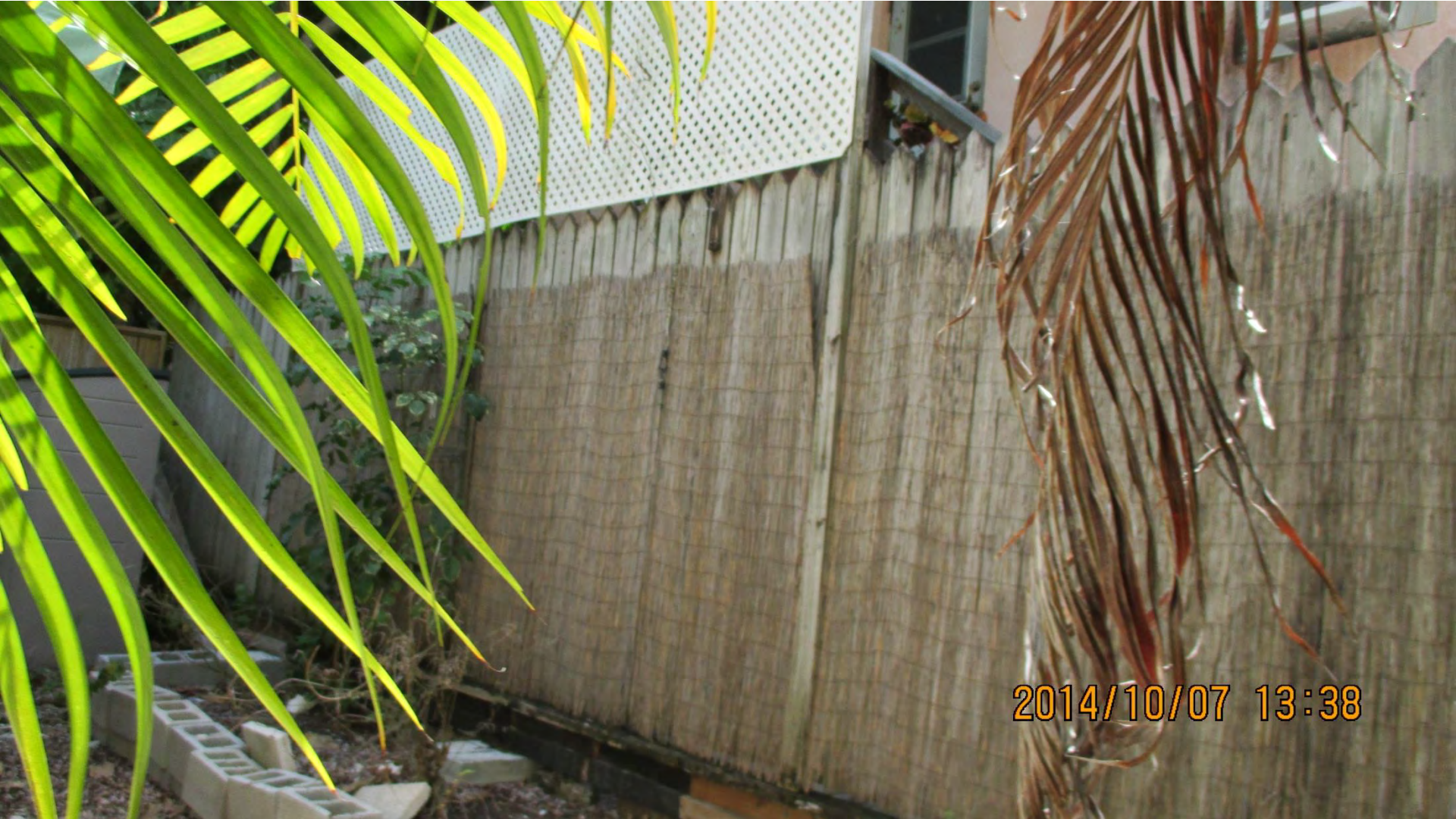
Rear of house where the deck is to be built.
