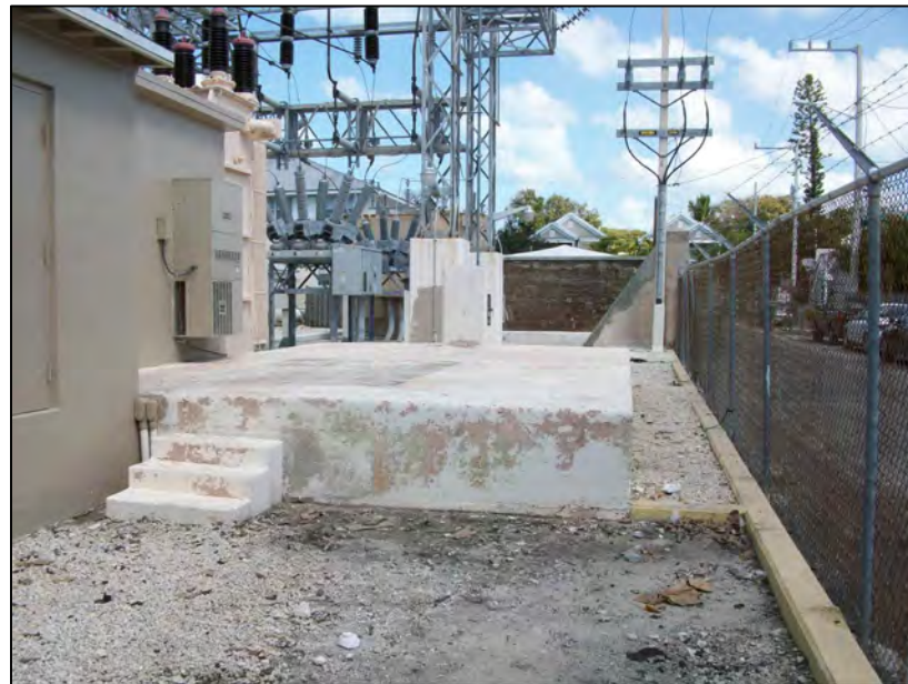
FOUNDATION TO BE REMOVED
