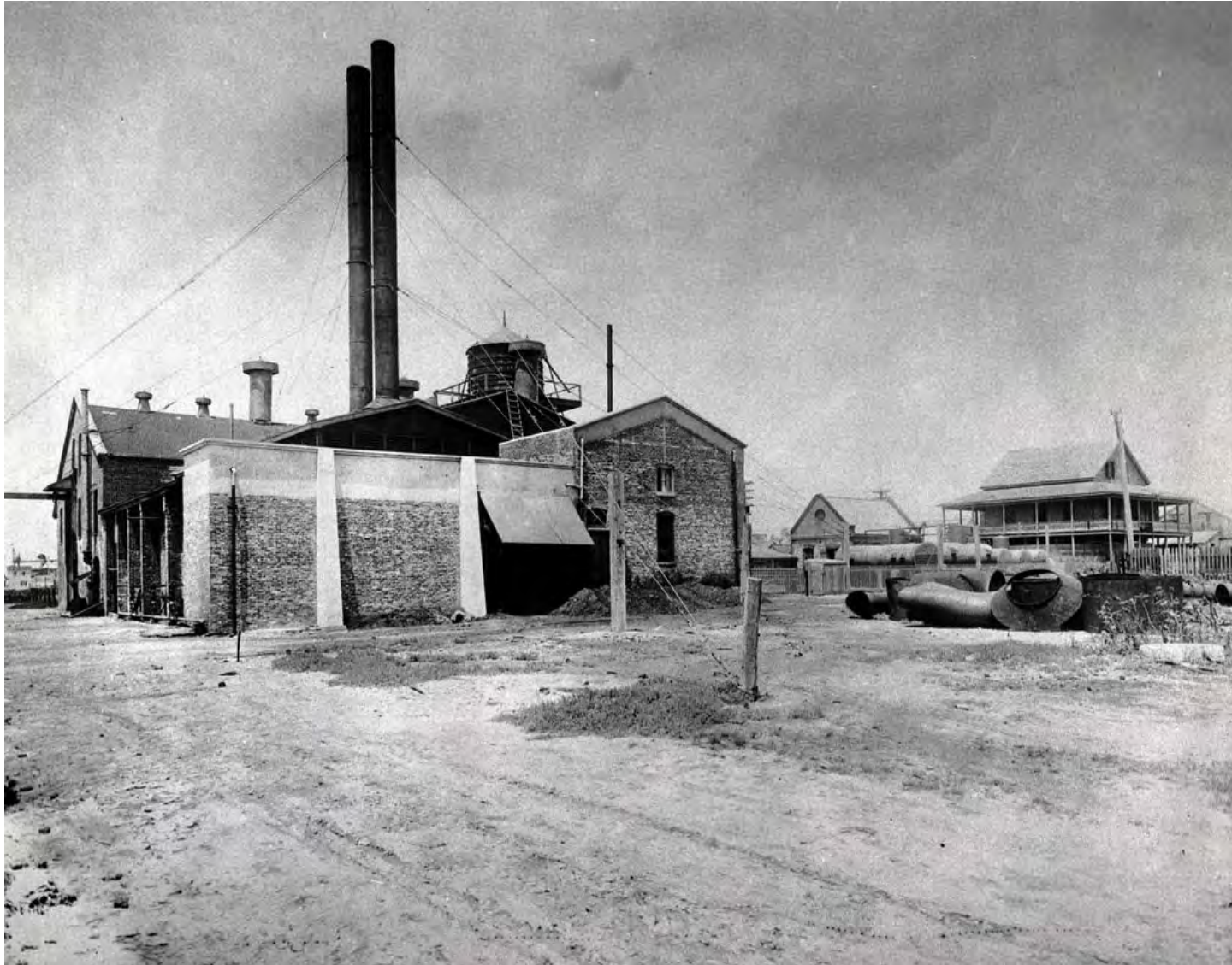
Key West Electric Plant ca.1900. Photograph taken from Fort Street. Photo from Monroe County Library Collection.
