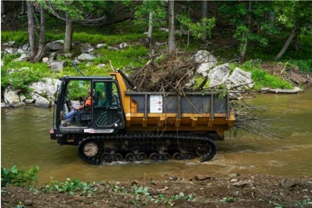
Visual reference: tracked equipment access for off-road and waterway-adjacent debris removal.
