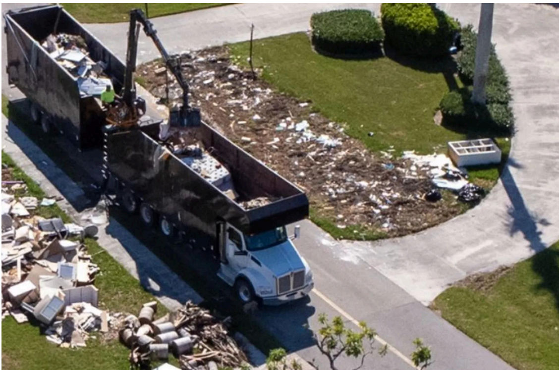
Curbside debris collection and grapple loading in dense residential conditions.
