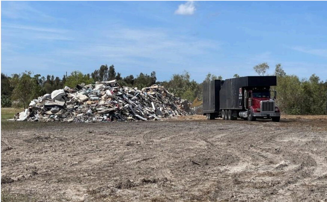
Visual reference: TOMS/DMS receiving and staging area with C&D-style debris stockpiling.
