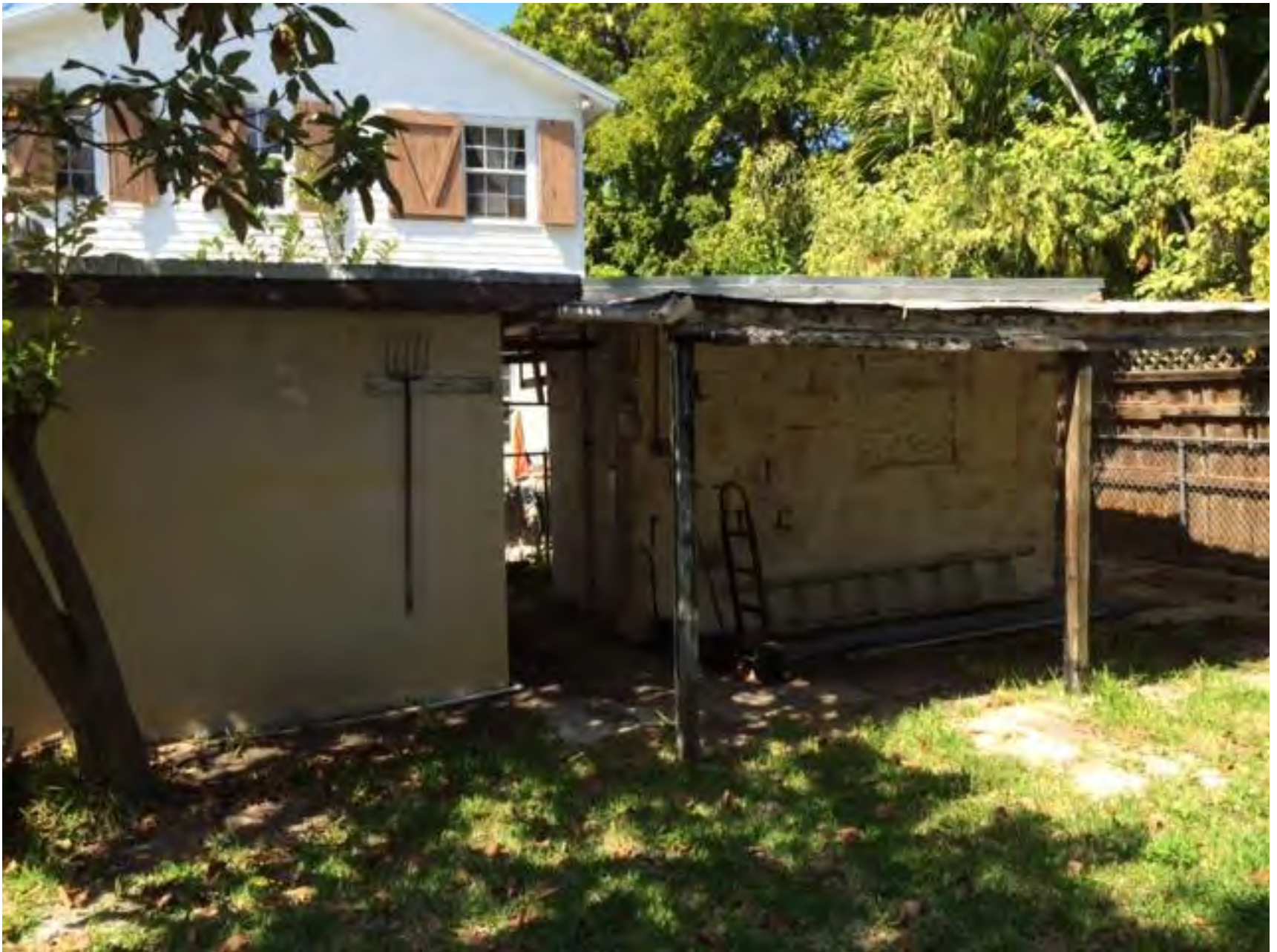
The two sheds at the rear of the property.
