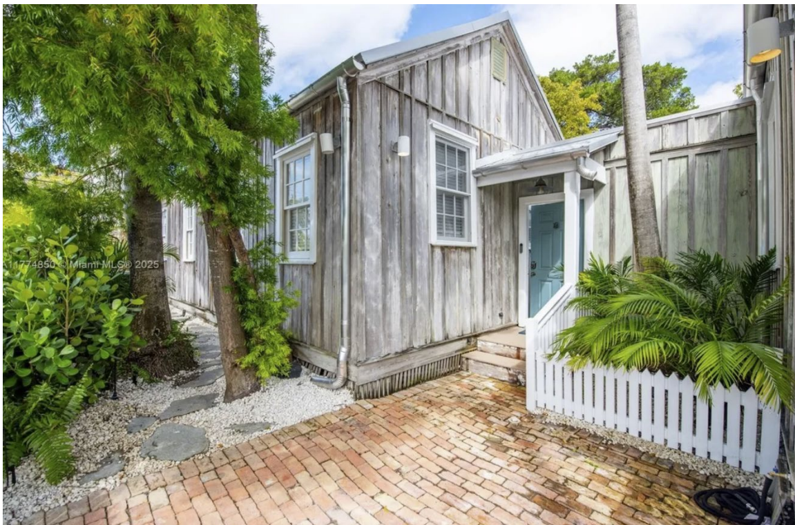
View of saloon wall and shed roof between two houses.
