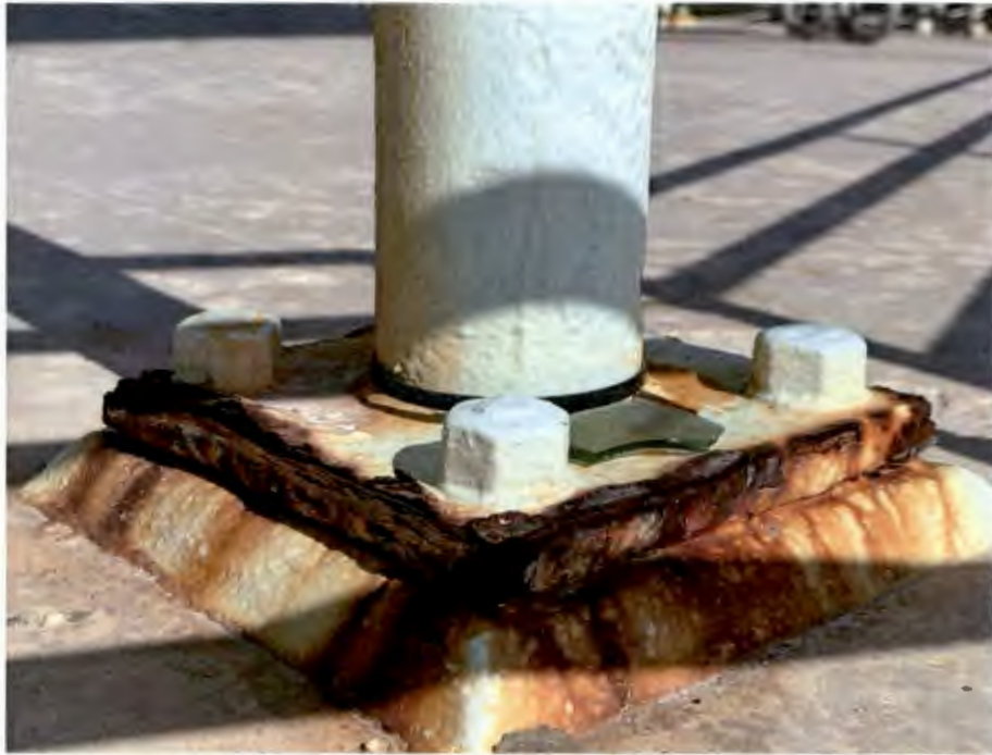
Figure 11 Painted and sealed anchor rod nut. Rust on edge of base plate which may be repaired.
