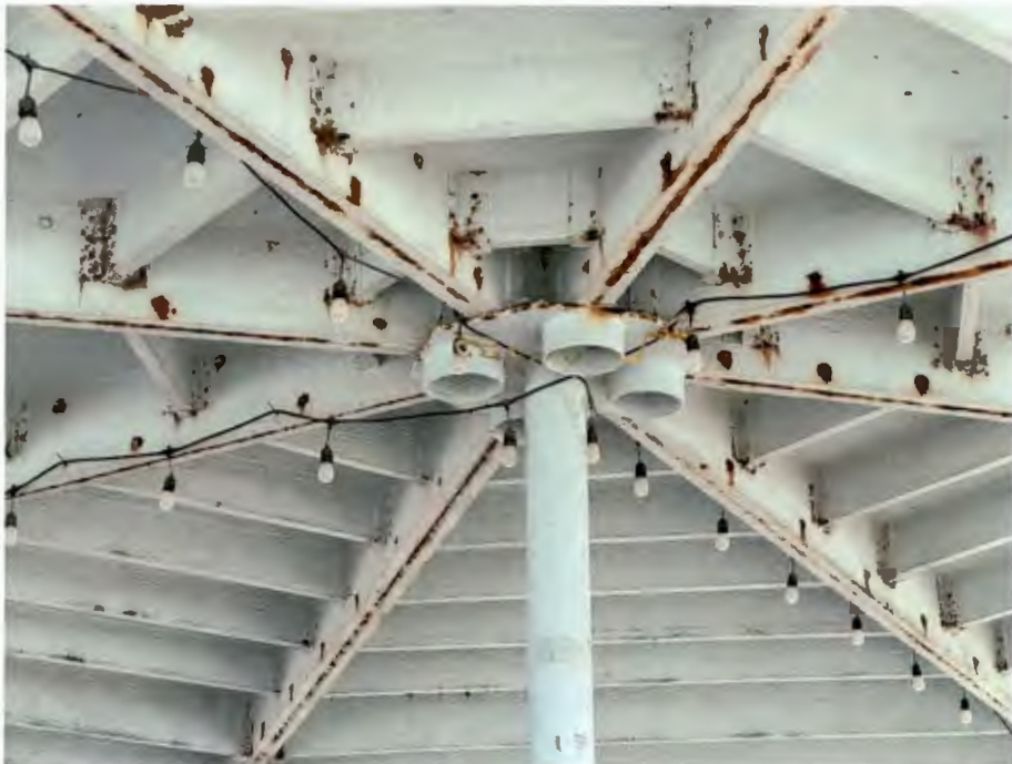
Figure 12 Rust visible at flitch beam plate and bolts.
