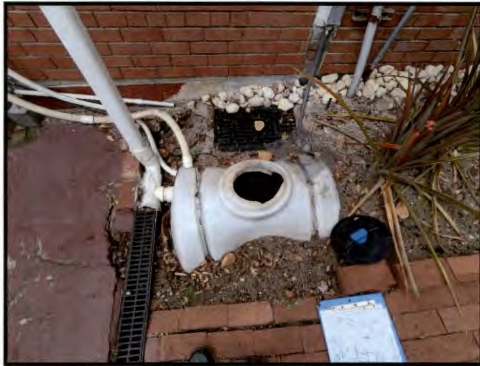
EXISTING 120 GALLON RAINWATER TANK
