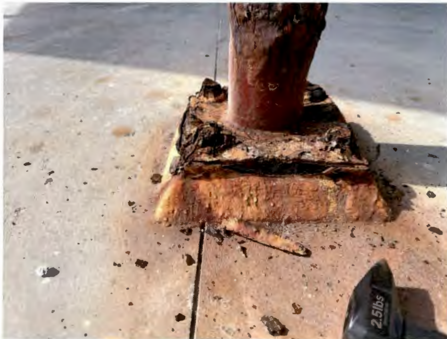
Figure 14 Deterioration at anchor rod nut which require replacement.
