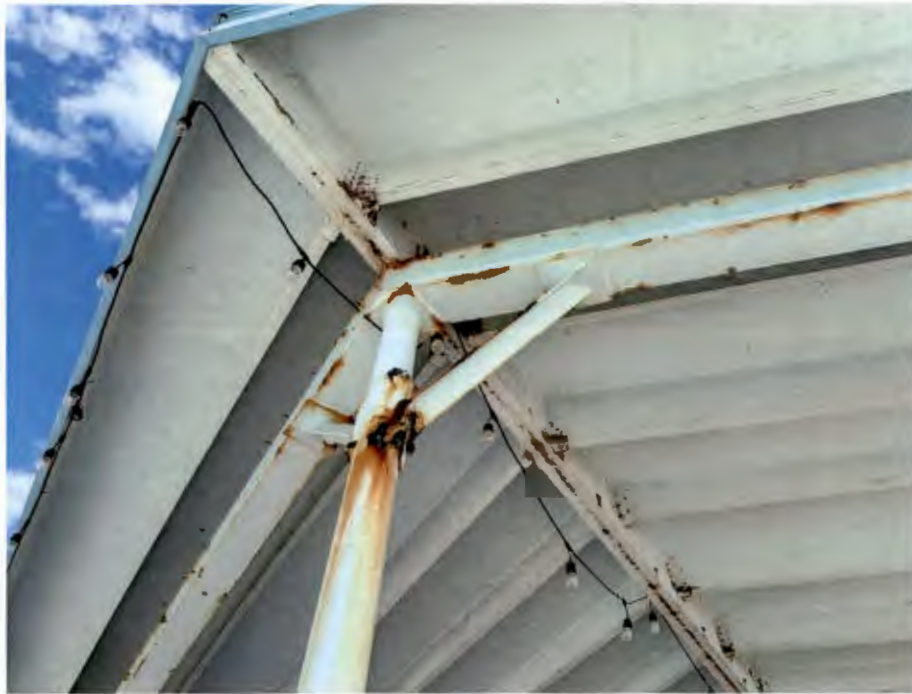
Figure 9 Rust at brace connection to post. Likely caused by water collecting on top of connection plate.
