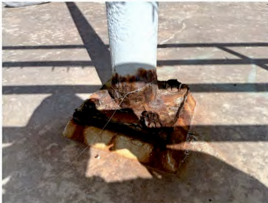
Figure 10 Deterioration of anchor rod nuts. Significant flaking.
