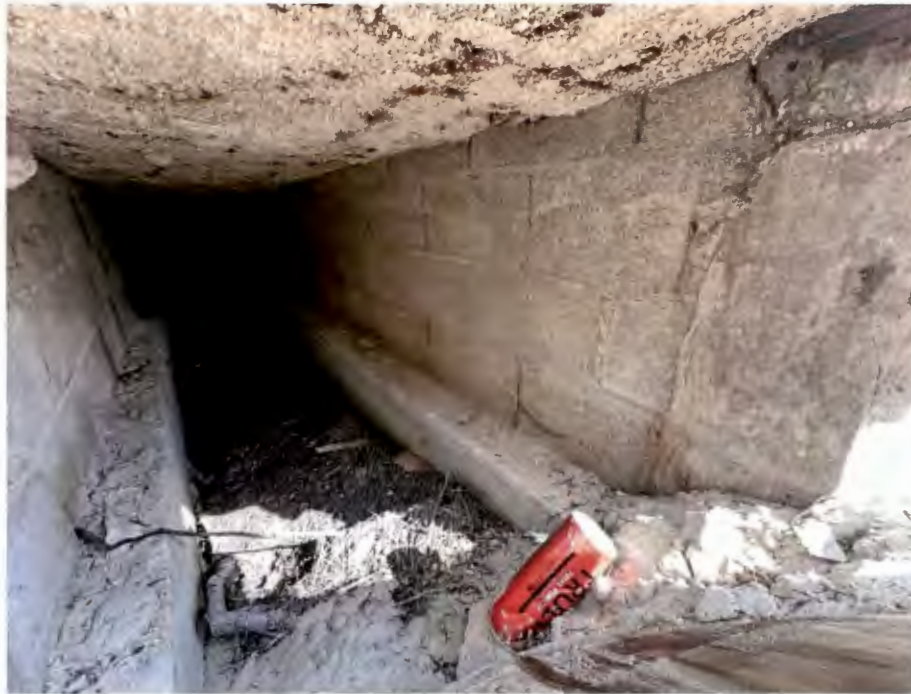
Figure 15 Wash out at ADA ramp of East pavilion.
