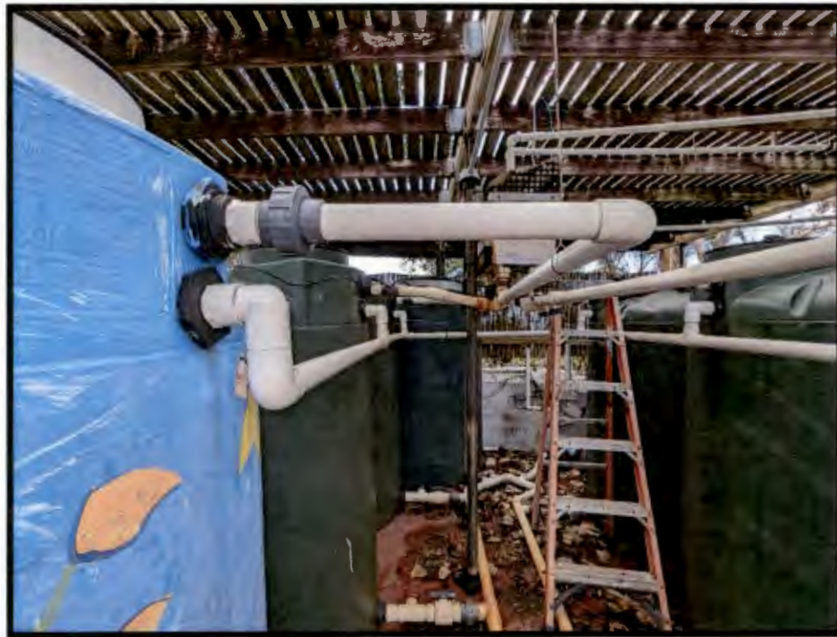
EXISTING SEVEN 500 GALLONS INTERCONNECTED IRRIGATION TANKS
