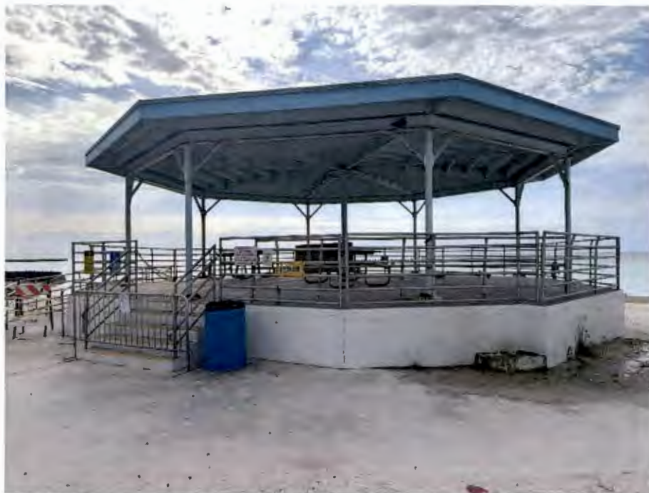
Figure 2 Overview of east pavilion from entrance. Note rust stains on beam flanges.
