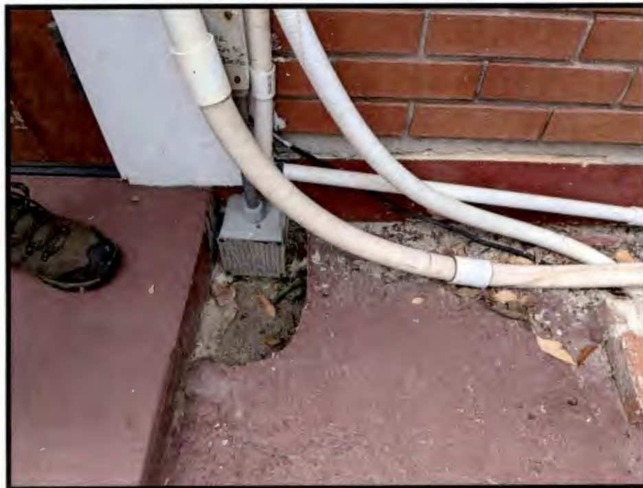
EXISTING PUMP#2 WATER LEVEL SENSOR
