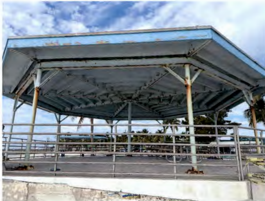
Figure 3 Rust on base plates, brace connections and beam flanges on east pavilion.
