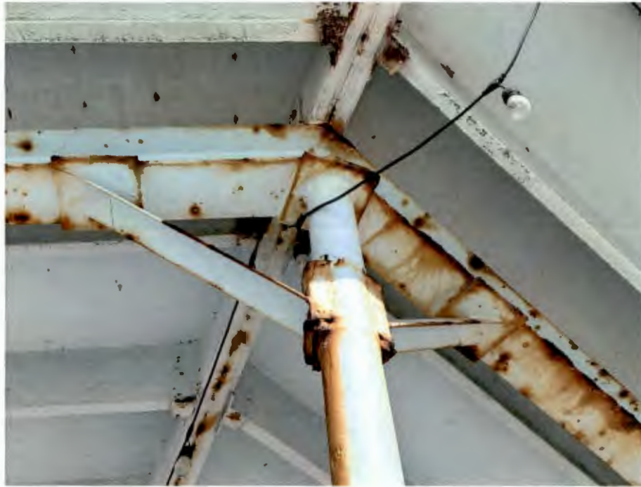
Figure 13 Rust at beam flanges and brace connections.
