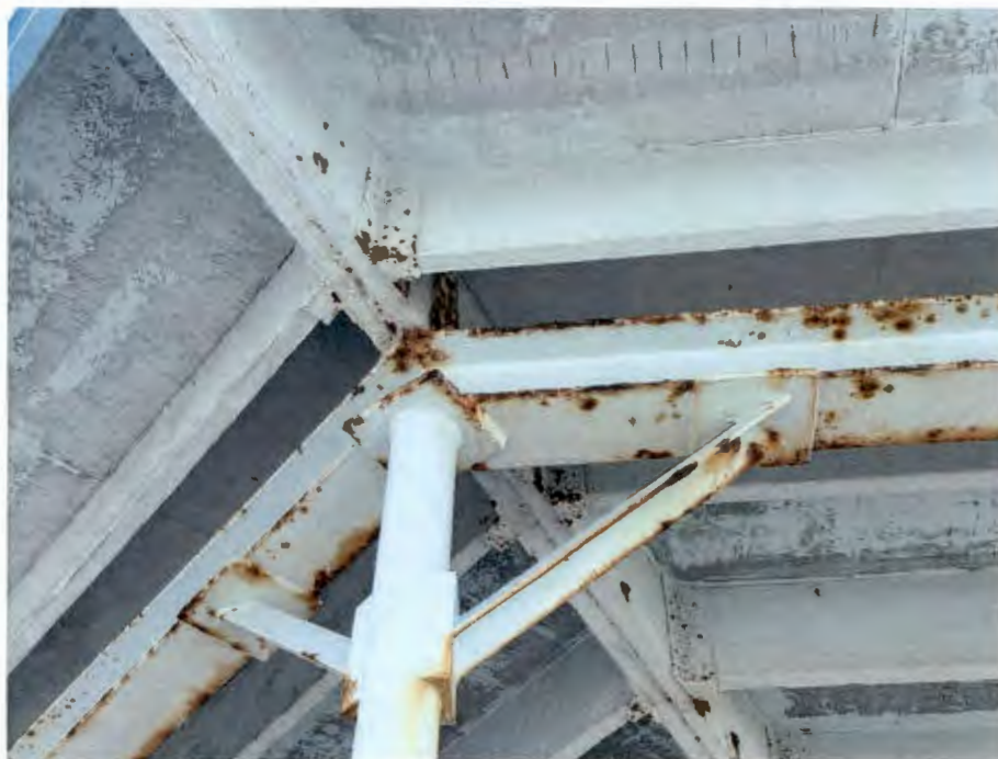
Figure 6 Rust spots along beam flanges and minor rust on rafter hangers.
