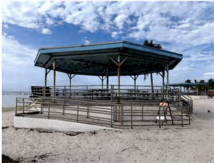
Figure 1 Overview of east pavilion. Note rust stains on posts.
