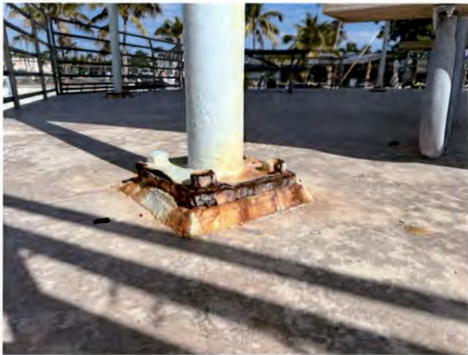
Figure 8 Base plate rusting and anchor rod.
