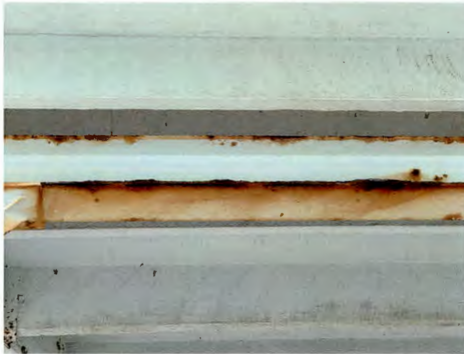
Figure 5 Rust at beam flange.
