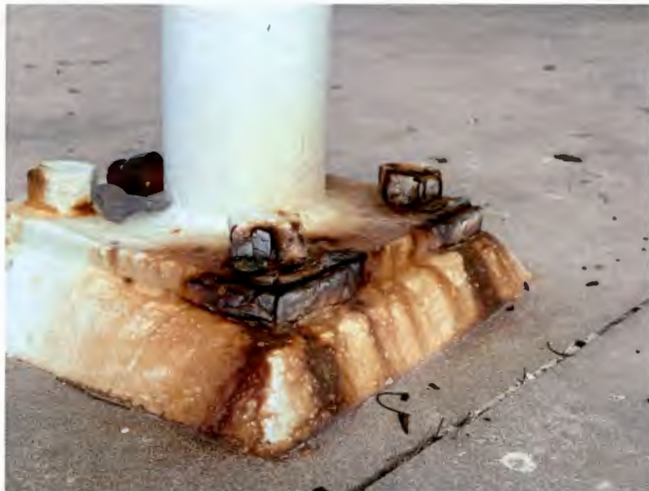
Figure 4 Rust on base plates and anchor rod nuts. Note flaking on nut.
