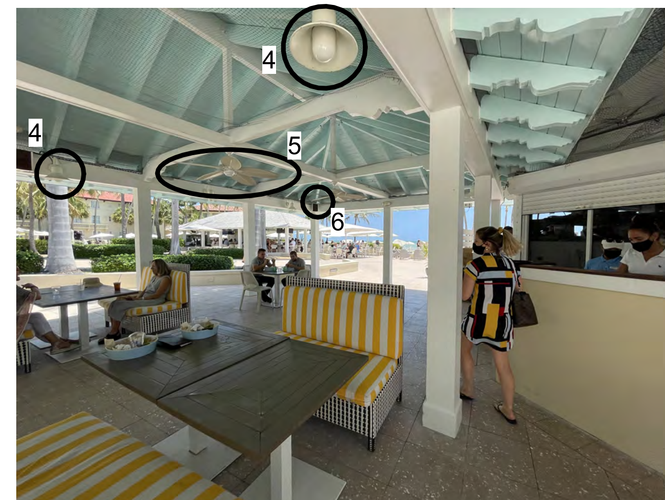
B1 REMOVE AND SALVAGE TO RETURN TO OWNER, TYPICAL THROUGHOUT SPACE 4. EXTERIOR LIGHTING 5. FANS 6. SPEAKERS
