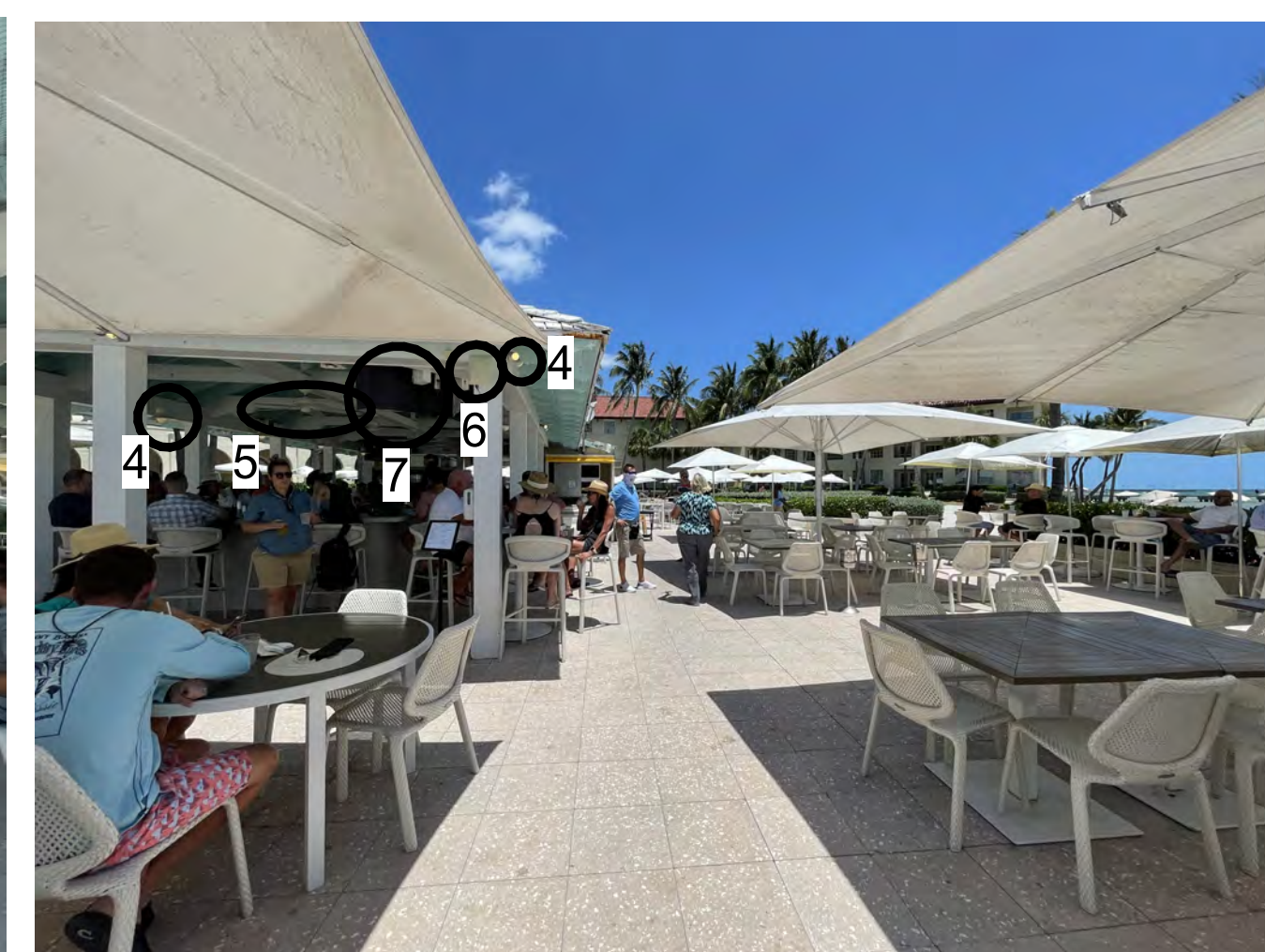
C REMOVE AND SALVAGE TO RETURN TO OWNER, TYPICAL THROUGHOUT SPACE 4. EXTERIOR LIGHTING 5. FANS 6. SPEAKERS 7. TVS
