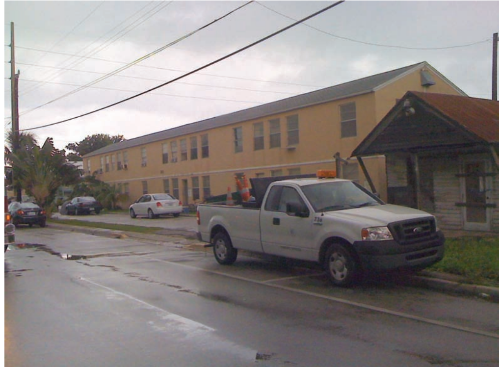
Roosevelt Sands Housing Authority residences slated for demolition
