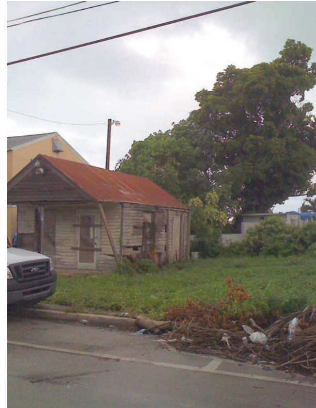
Vacant lot & deteriorated building across Emma Street
