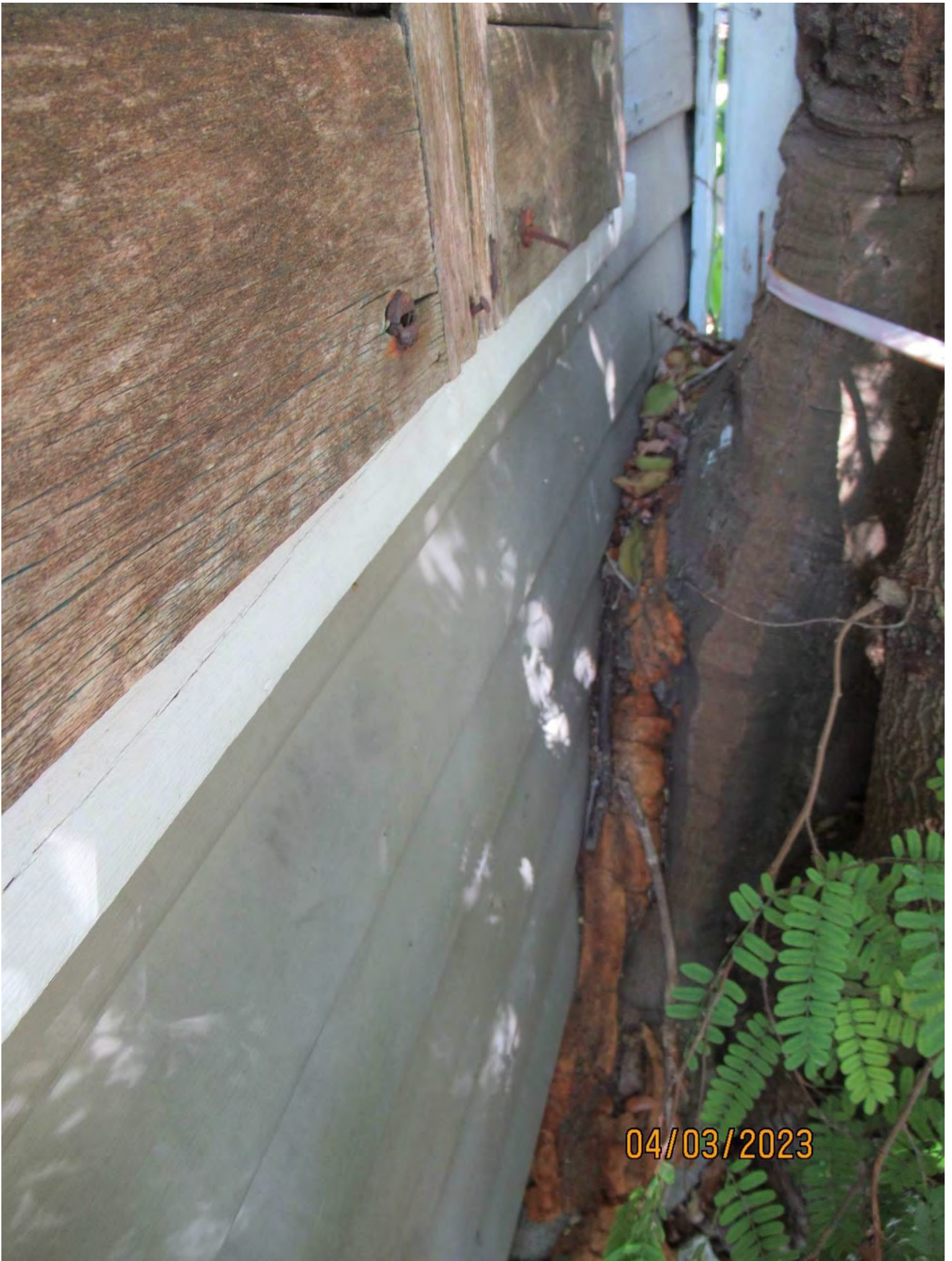
Photo of tree trunk in relation to historic structure, view 3.
