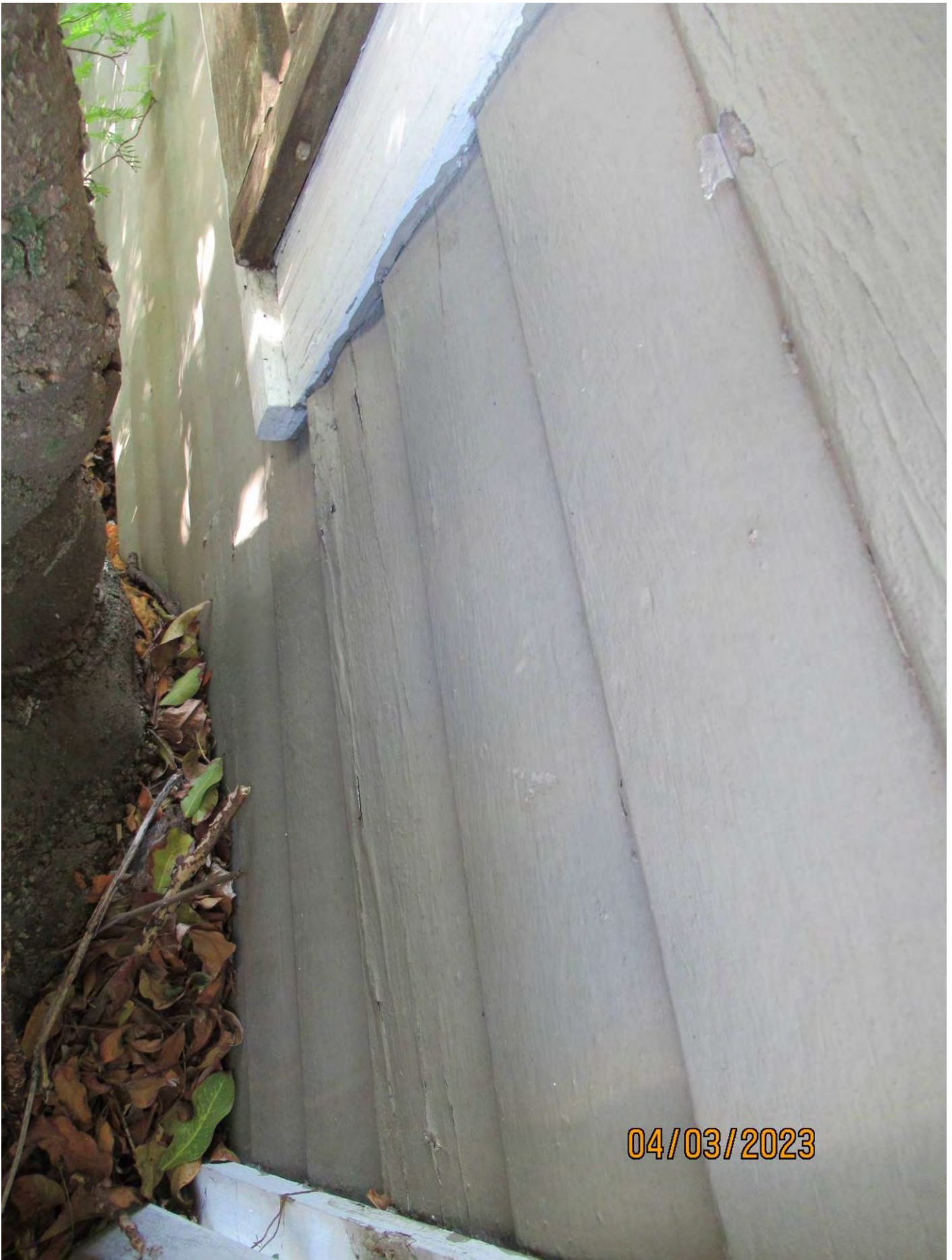
Photo of tree trunk in relation to historic structure, view 1.
