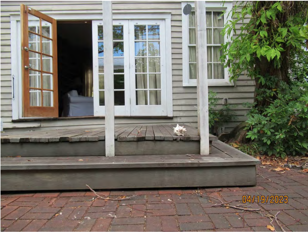
Photo showing location of tree in relation to raised floor area.
