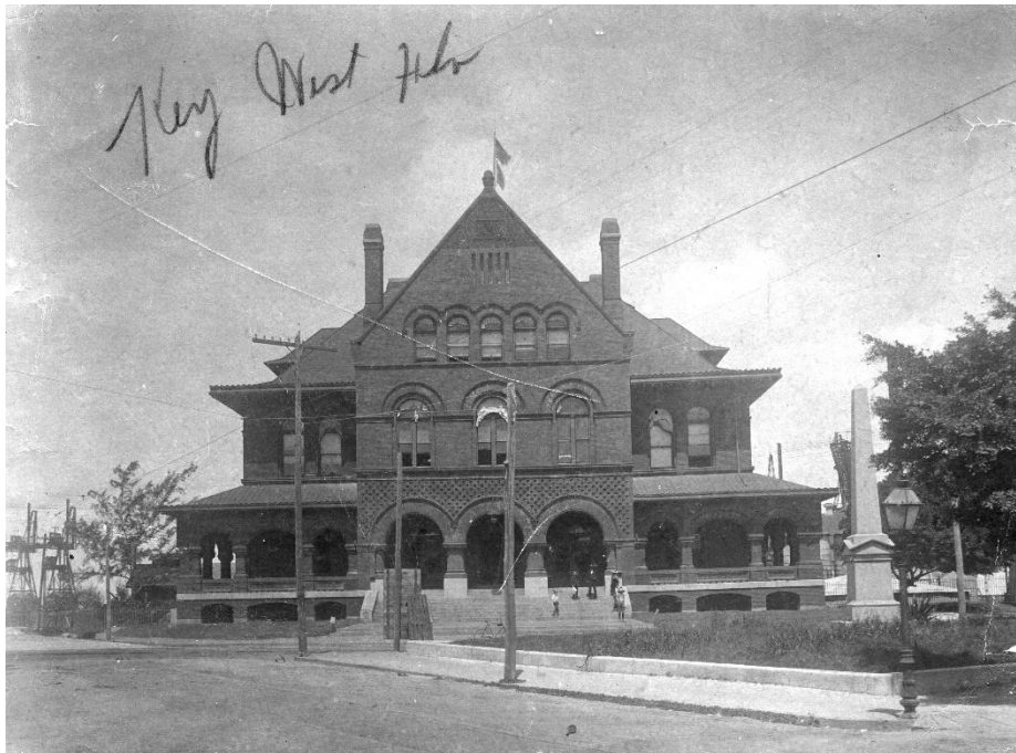
Clinton Square and Custom House circa 1890's. Monroe County Library.
