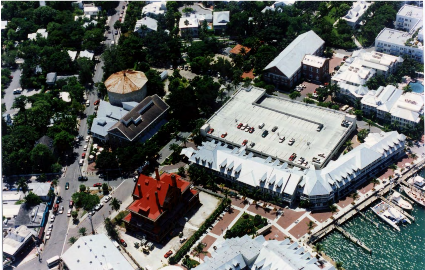
Aerial 1999. Monroe County Library.
