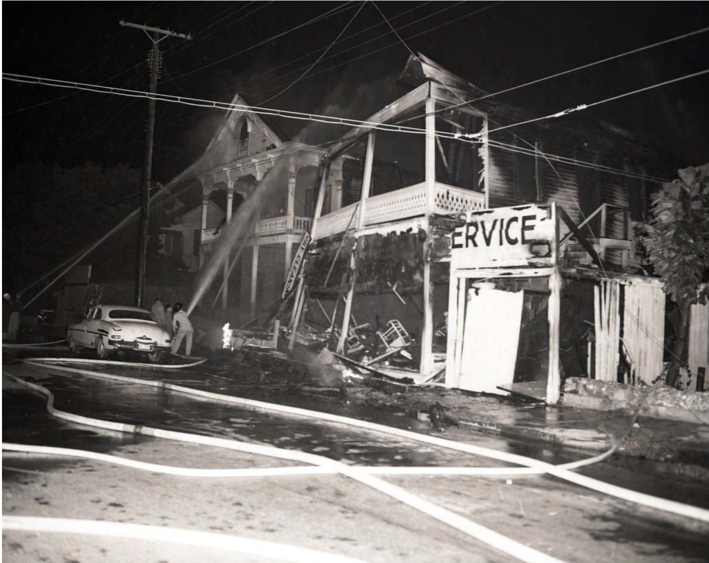
218 Simonton Street on October 29, 1957, after fire destroyed the two-story building that housed the Poinciana Laundry. Monroe County Library.
