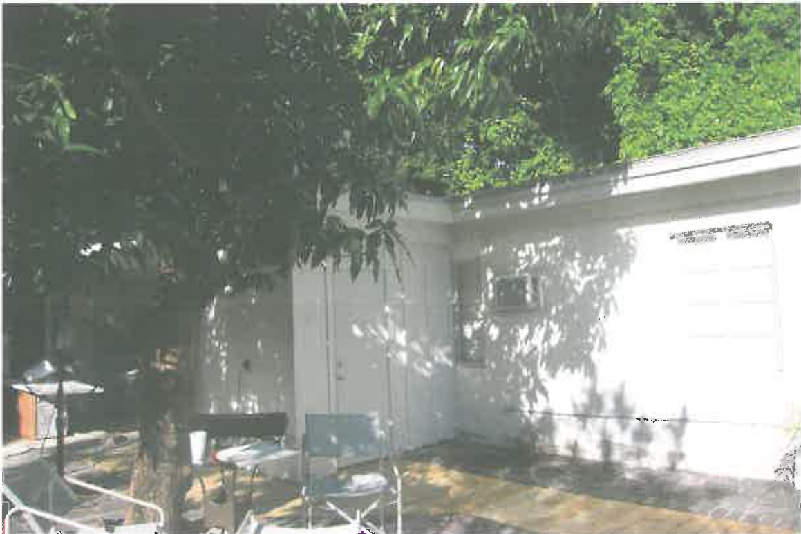
EXISTING BUILDING ON SITE
