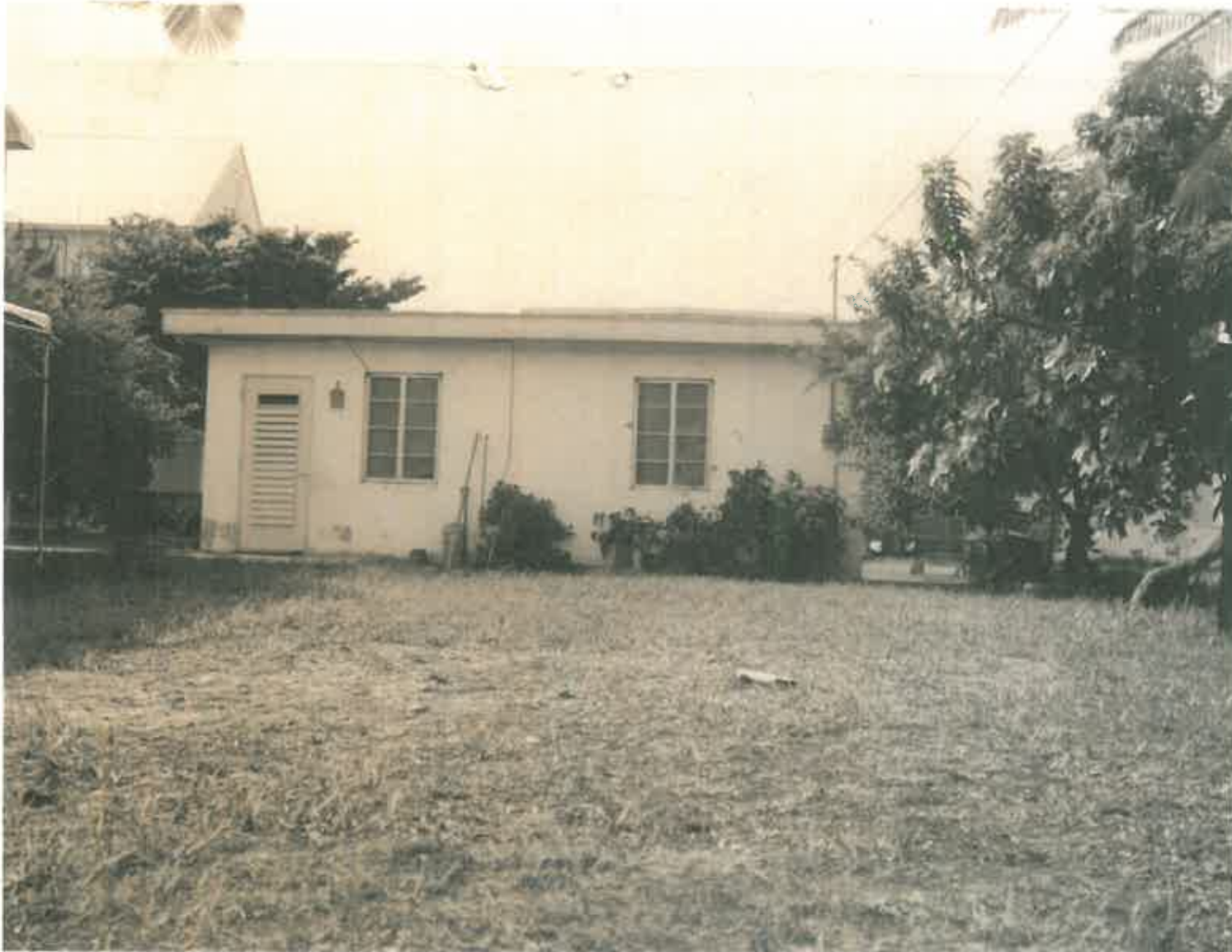
Photo taken by Property Appraiser's office c1965; 907 Eaton St. Monroe County Library
