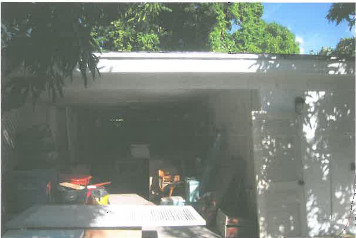
EXISTING BUILDING ON SITE
