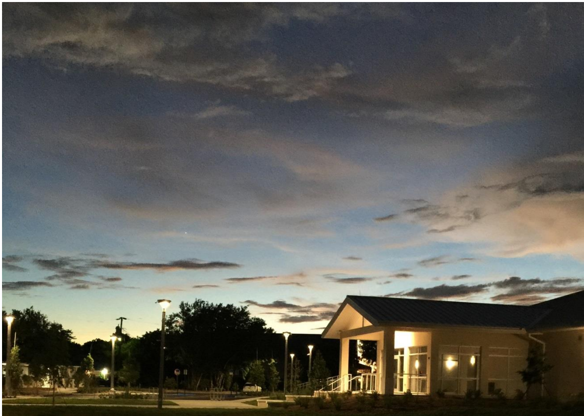
Recent Electrical Work - Parking Lot Lighting at Marathon City Hall
