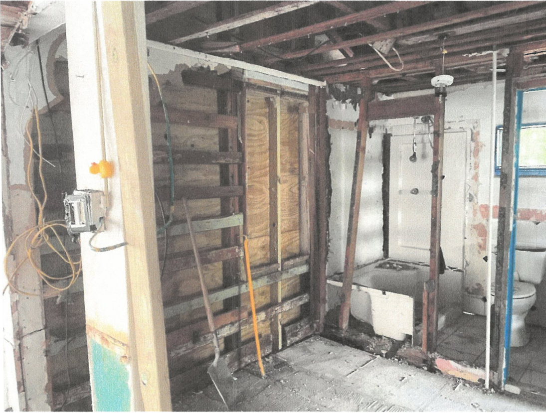
Photograph 2: Interior of the structure.
