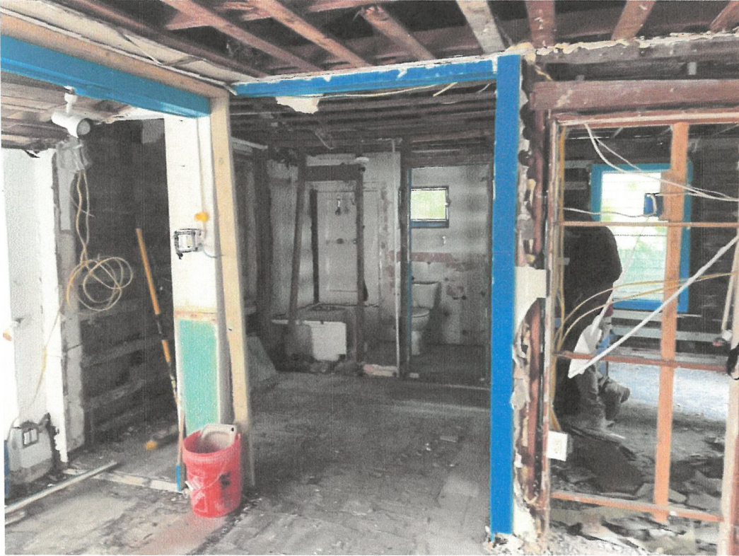
Photograph 3: Another picture of the interior of the structure.
