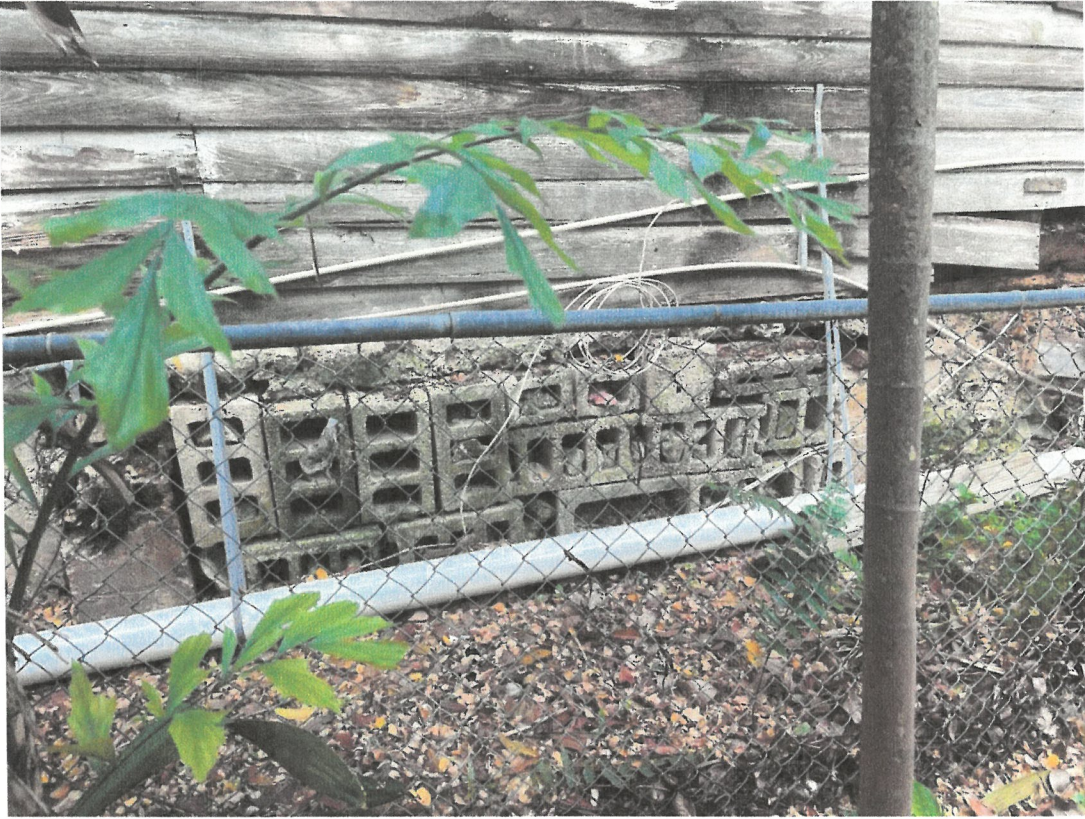
Photograph 6: Another photograph showing the foundation. .
