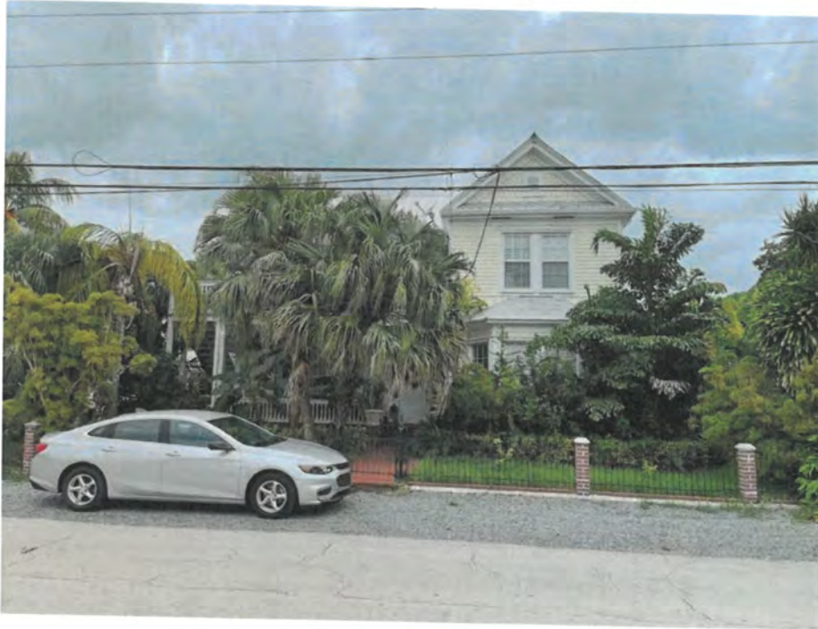
Figure 1 – South view of existing residence
