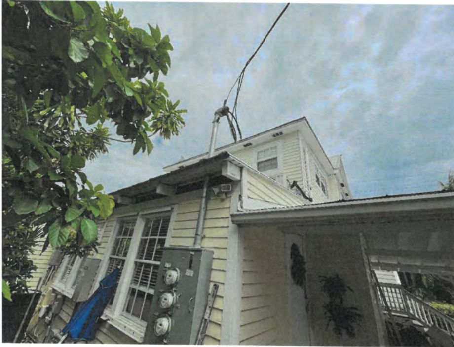
Figure 7 – North view of existing residence
