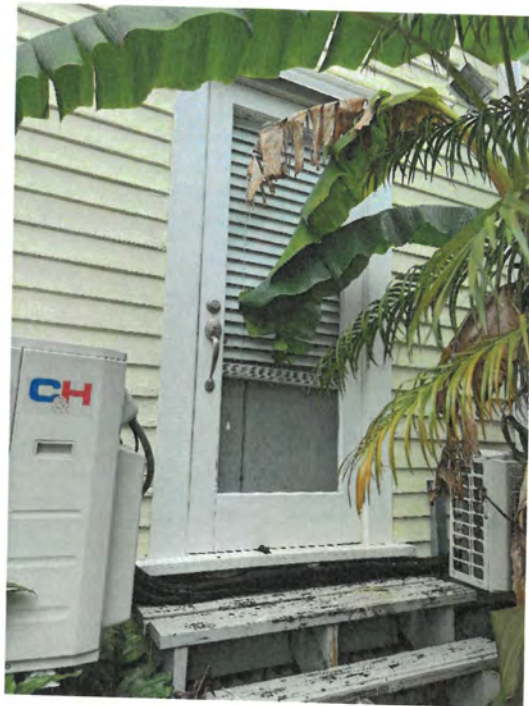
Figure 12 – Door on east side of existing residence, to be removed
