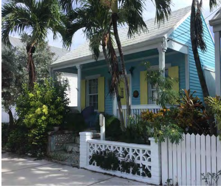
718 Southard Street prior to demolition.
