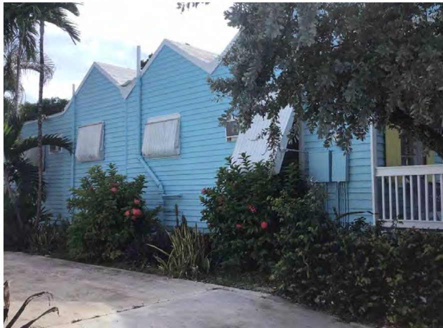
718 Southard Street prior to demolition.
