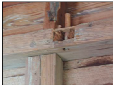
Exposed mortise & tenon construction techniques typical of the period
