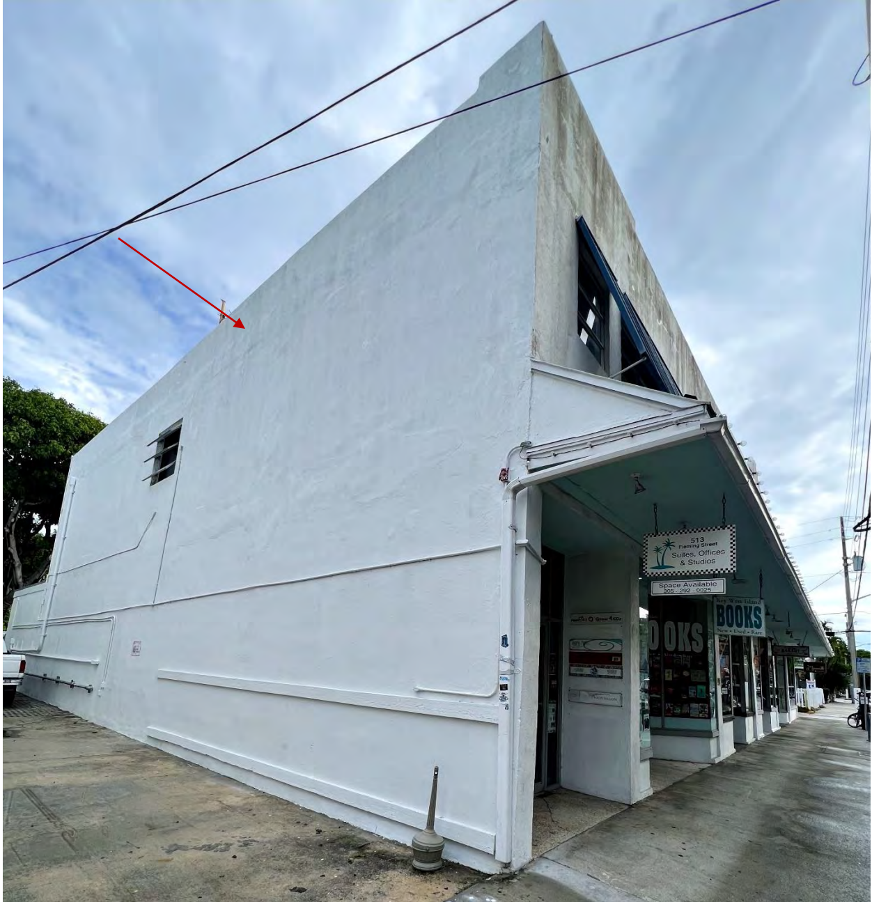
Wall under review.
