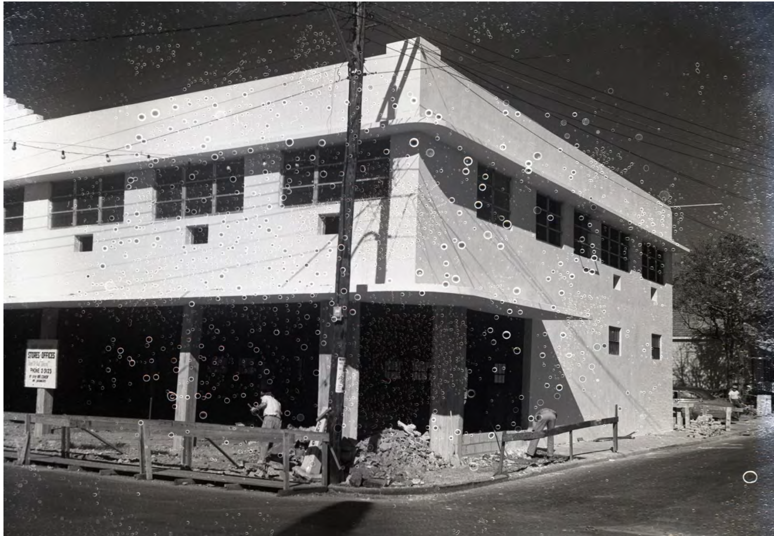
513-521 Fleming Street under construction in February 1954. Monroe County Library.
