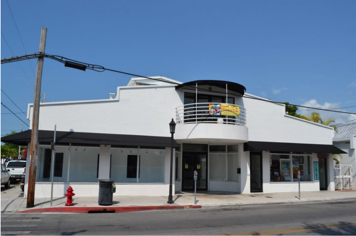
Photo of property under review 2011, view from Duval Street.
