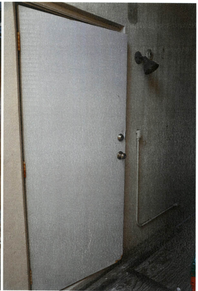
SIDE EXIT DOOR
