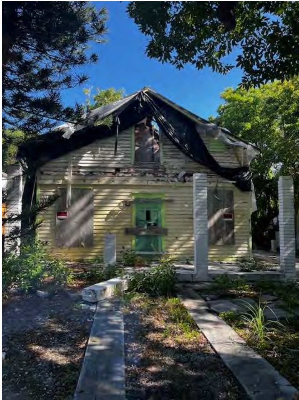
The house before demolition.
