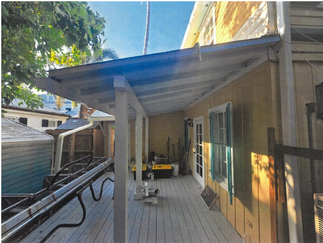
Photo of Rear Covered Porch Proposed to be Enclosed.
