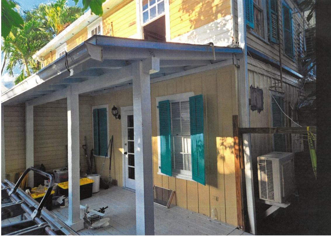
Photo of Rear Covered Porch Proposed to be Enclosed
