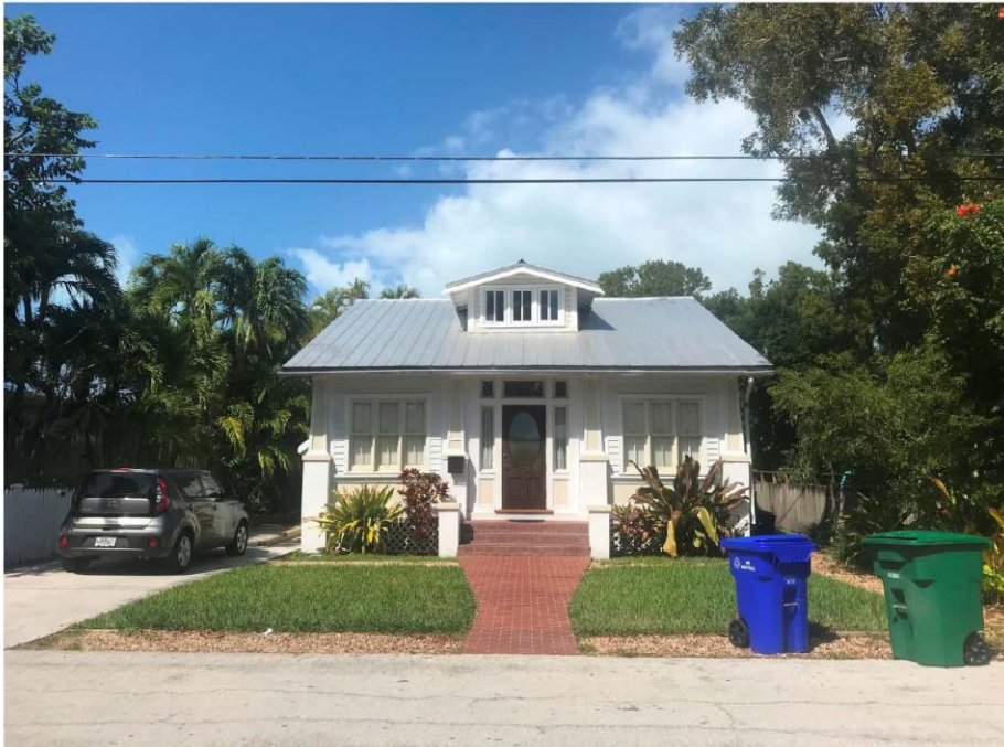
1217 WASHINGTON STREET LEFT NEIGHBORING PROPERTY FRONT VIEW
