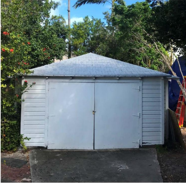
1227 WASHINGTON STREET GARAGE FRONT VIEW
