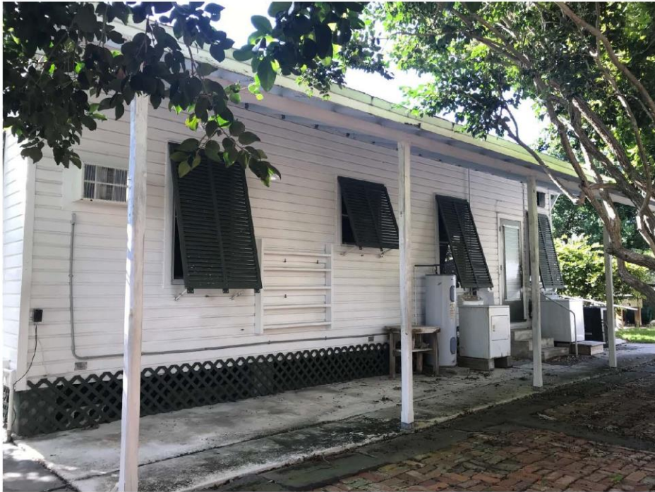
1227 WASHINGTON STREET REAR VIEW
