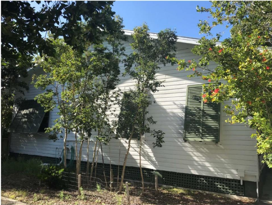
1227 WASHINGTON STREET SIDE VIEW
