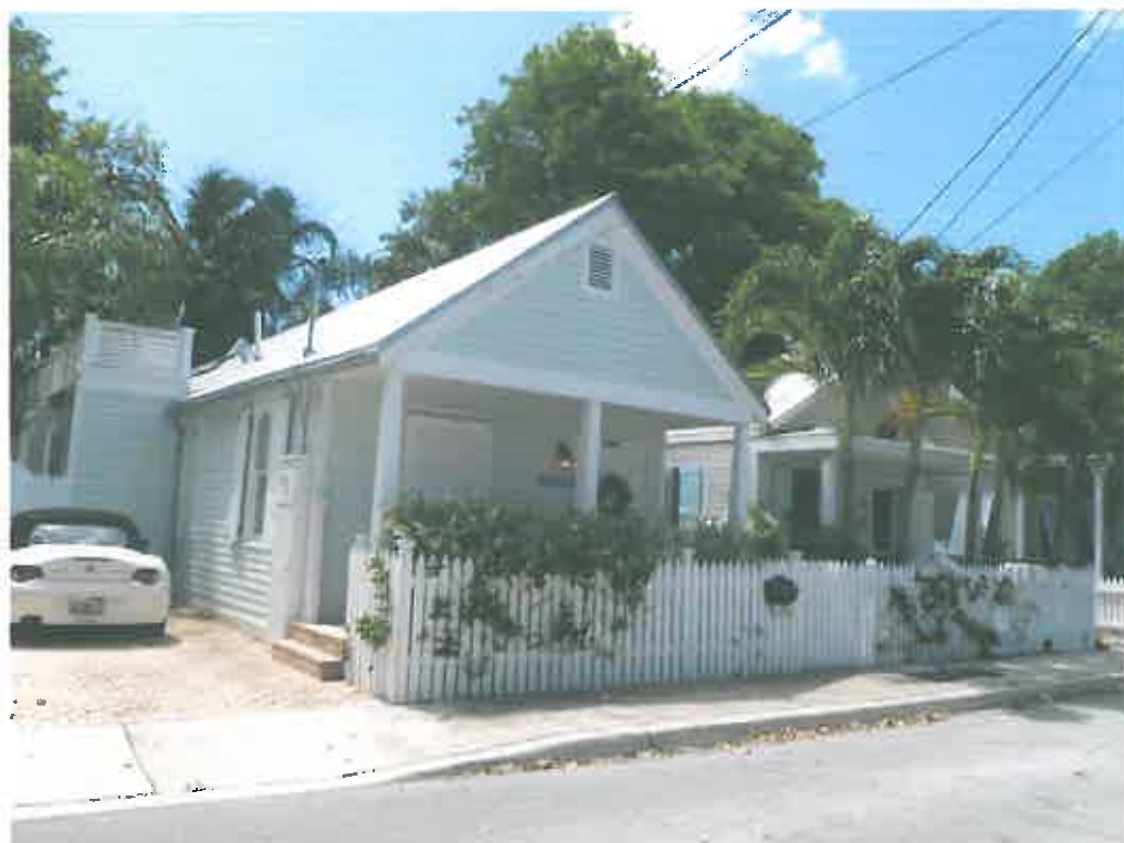
414 Louisa Street - Adjacent Property
