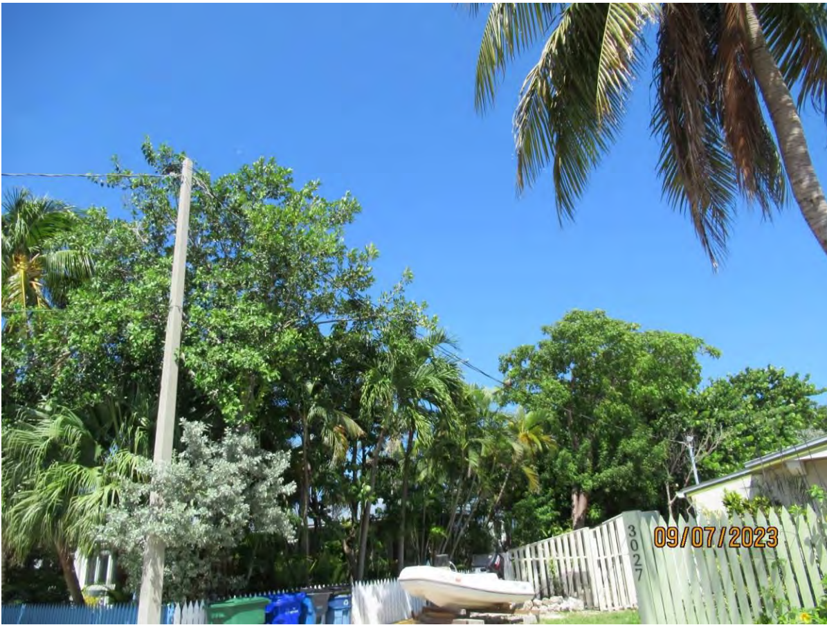
Photo showing electrical lines and tree canopy.
