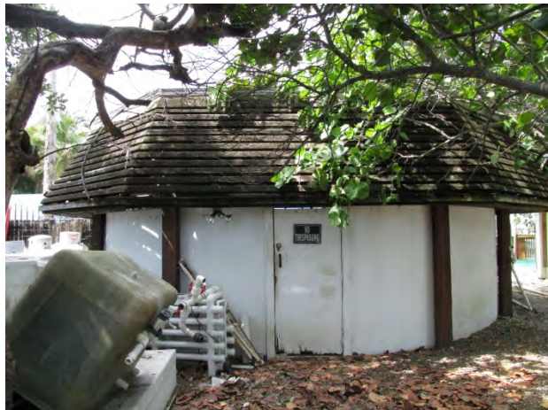
Mallery Square East Cable Hut, as seen from Mallery Square. This structure is currently used as a pump room for the Key West Aquarium.
