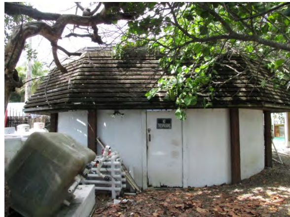
The exterior of the east Cable Hut. The heavy timber columns can be seen spaced around the tank. The door is the only entry into the East Cable Hut.
