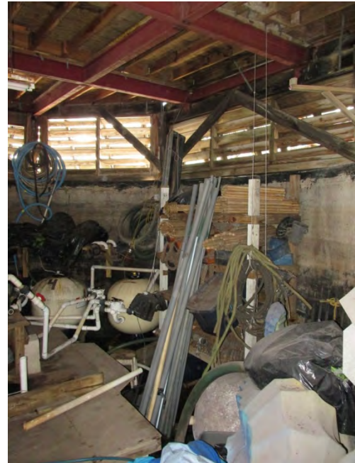
Interior view of the East Cable Hut. The space is littered with shelving, unused equipment, pumps, piping, and wiring.
