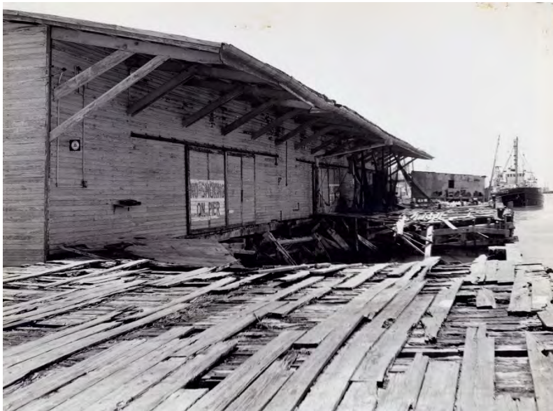
This famous view of the Mallory Docks was taken by photographer Don Pinder in 1961. The Mallory docks are severely deteriorated. The warehouse was originally operated by the Mallory Steamship Line. The Cable Huts are located just beyond the warehouse building. This warehouse building would be demolished soon after this photo was taken.
