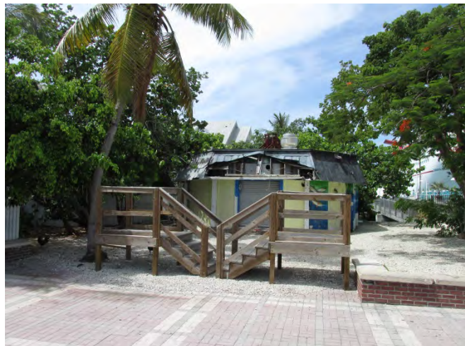
A view of the Cable Huts from Mallory Square. Mallory Square is paved in attractive brick, with accent walls and light fixtures, but the site work does not extend to the area around the Cable Huts. Instead, a set of temporary stairs blocks access to the area.
