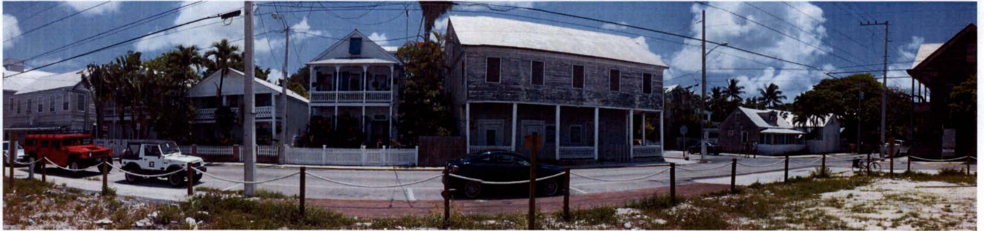
⊕ VIEW LOOKING AT CAROLINE STREET FROM PROPERTY
