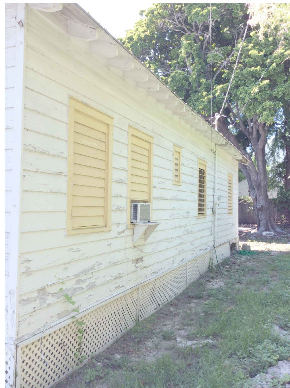
FIGURE 4 RIGHT SIDE VIEW OF HOUSE
