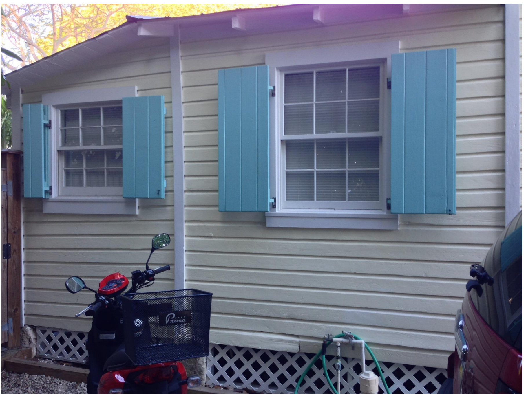
Close-up of the two rear additions; east elevation.
