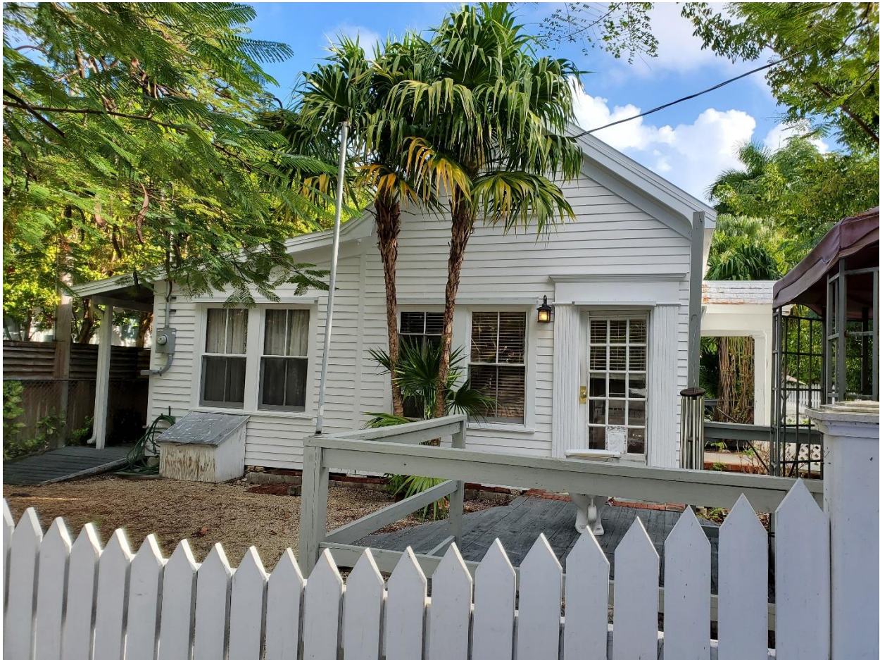
View of West Elevation from Outside Property
